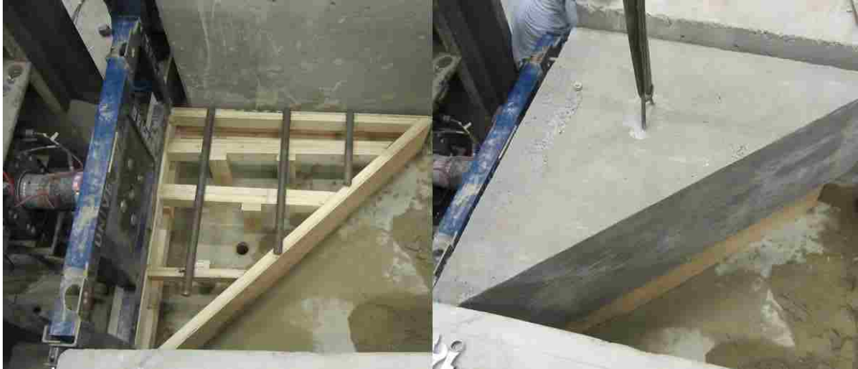
Figure 3-2: Photographs Taken During Placement of 45° Backwall
