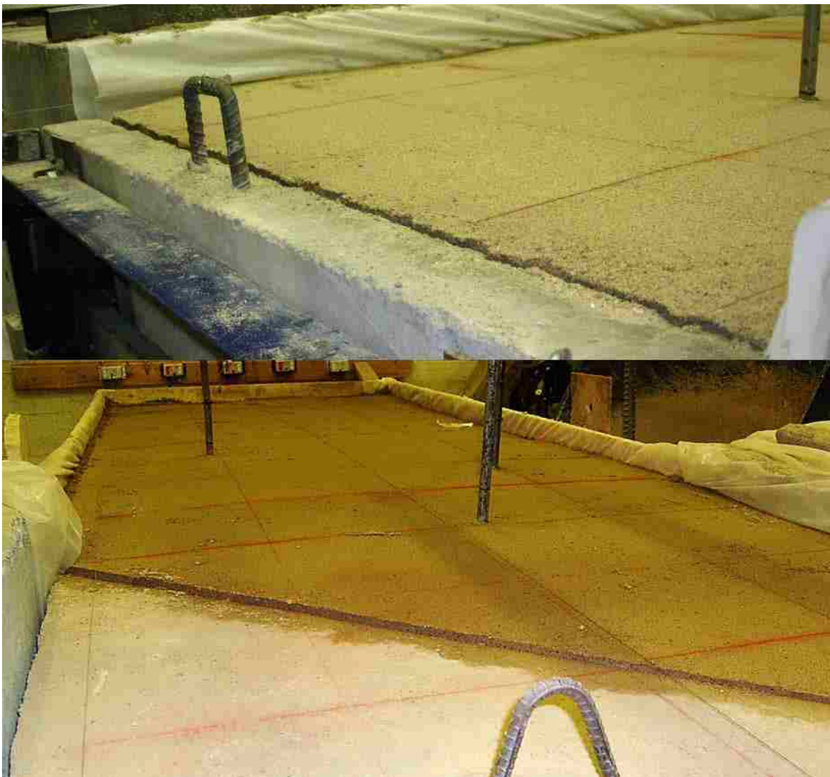
Figure 4-16: Photos of Ground Surface Heave near the Backwall for both a Non-Skew and 45° Skew Test
