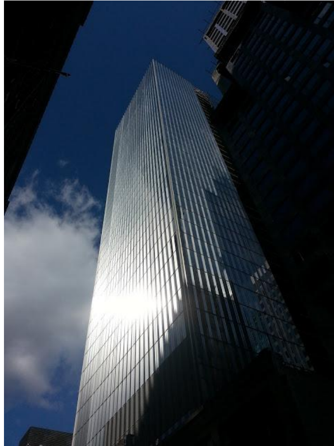
Figure 7 - 250 West 55th Street Building
