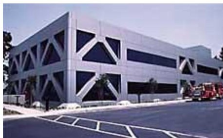
Figure 13 - Los Angeles Fire Department Control Facility
