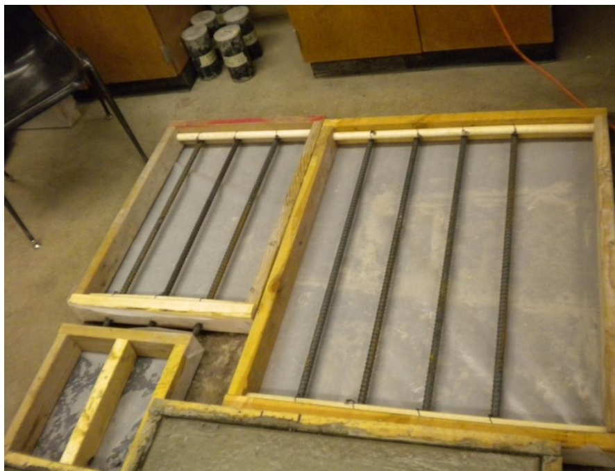
Figure 3-5: Forms prepared for concrete slabs.
