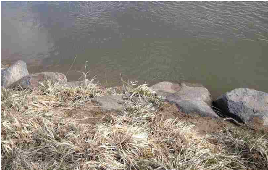
Figure 3-7: Tight Vane Angle Protected and Stabilized the Streambank. Flow from Right to Left (Picture Taken by Evan Cope).
