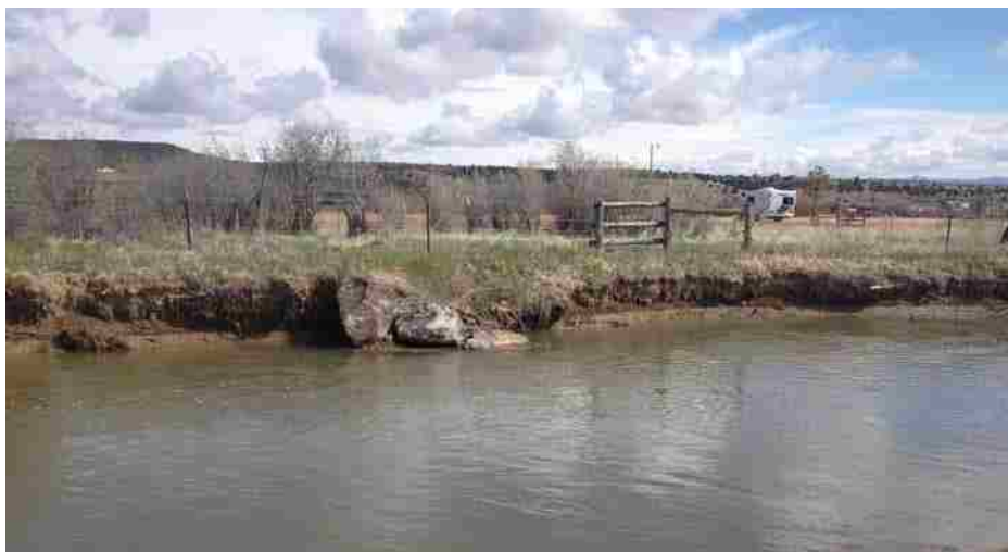
Figure 3-5: Large Vane Angle that Created a Recirculating Eddy and has Actually Increased Streambank Erosion. Flow from Right to Left. (Picture taken by Evan Cope).
