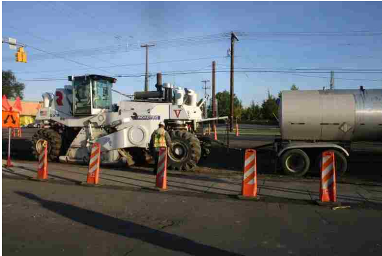
Figure 2-2: Asphalt emulsion injection at 7800 South.
