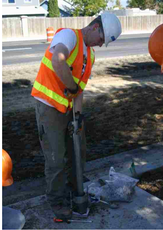
Figure 3-3: Compaction of emulsion-treated base specimen at 7800 South.
