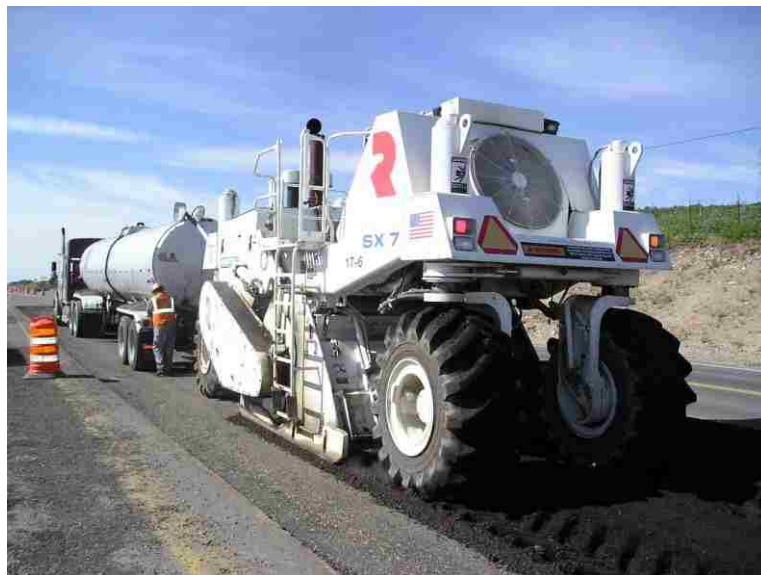
Figure 2-1: Asphalt emulsion injection at Redwood Road.
