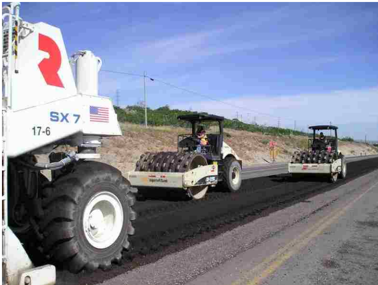
Figure 2-3: Compaction of emulsion-treated base layer at Redwood Road.
