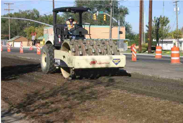
Figure 2-4: Compaction of emulsion-treated base layer at 7800 South.
