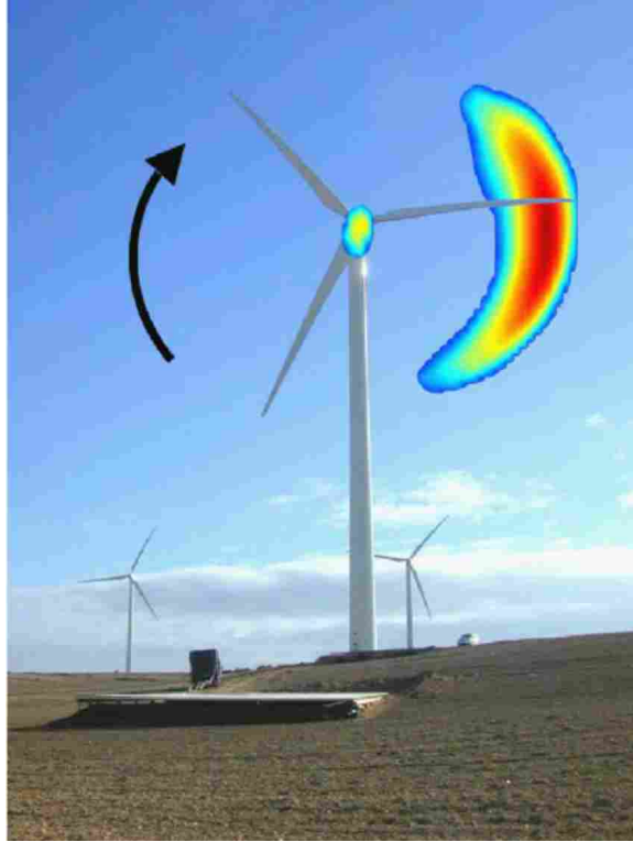
Figure 1.4: An illustration of a G58 wind turbine with an averaged acoustic distribution of the blades projected on the picture, taken from the work of Oerlemans et al. [4]
