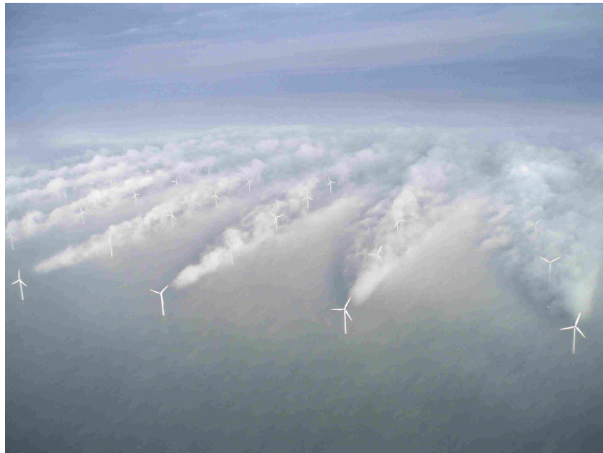
Figure 1.3: An example of wind turbine wake interference from Horns Rev Wind Farm in Denmark. (Christian Steiness/Vattenfall, “Horns rev offshore wind farm,” January 13, 2010 via Flickr, Creative Commons Attribution)
