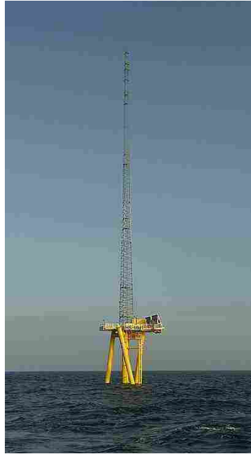
Figure 1.3: Demonstration of the IBGS at Hornsea [58].
