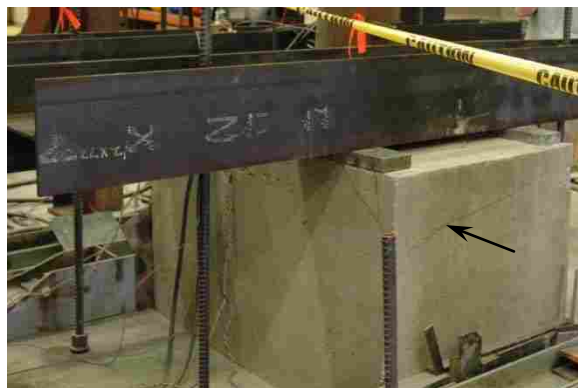
Figure 4-11: Cracking at the End of Specimen 3 (North-South)
