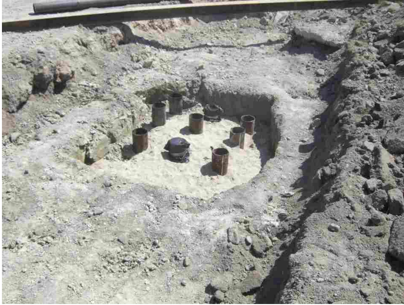
Figure 4-2 Driven pile layout prior to cap construction.
