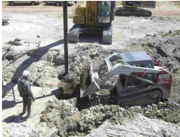
Figure 5-1 Placement of 1 ft lift for compaction of main body of RAP
