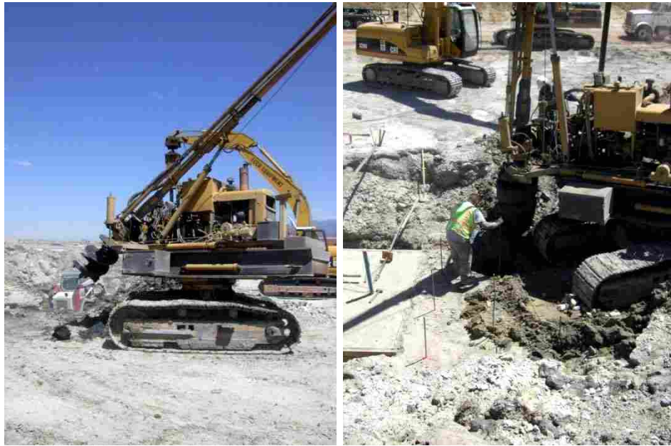
Figure 5-7 Excavation for RAP installation
