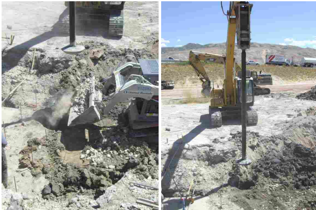
Figure 5-8 Ramming of base material into bottom of excavated RAP hole
