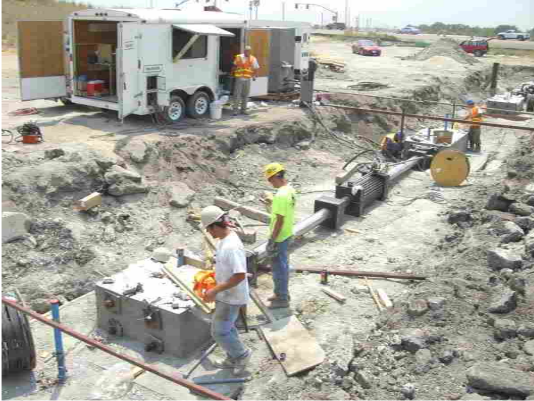
Figure 4-9 Photo of actuator setup between caps 1 & 2
