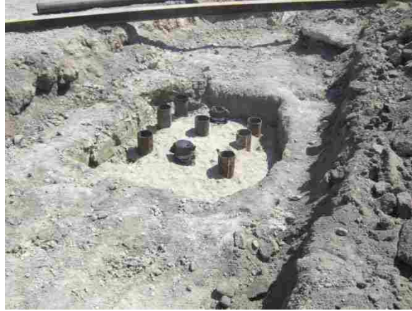
Figure 4-3 Driven pile layout prior to cap construction
