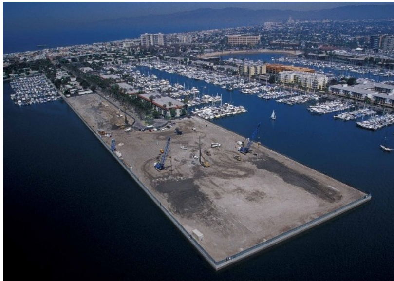
Figure 5-1 Esprit Apartments site, Marina del Rey, CA (source, Hayward Baker, Inc.).
