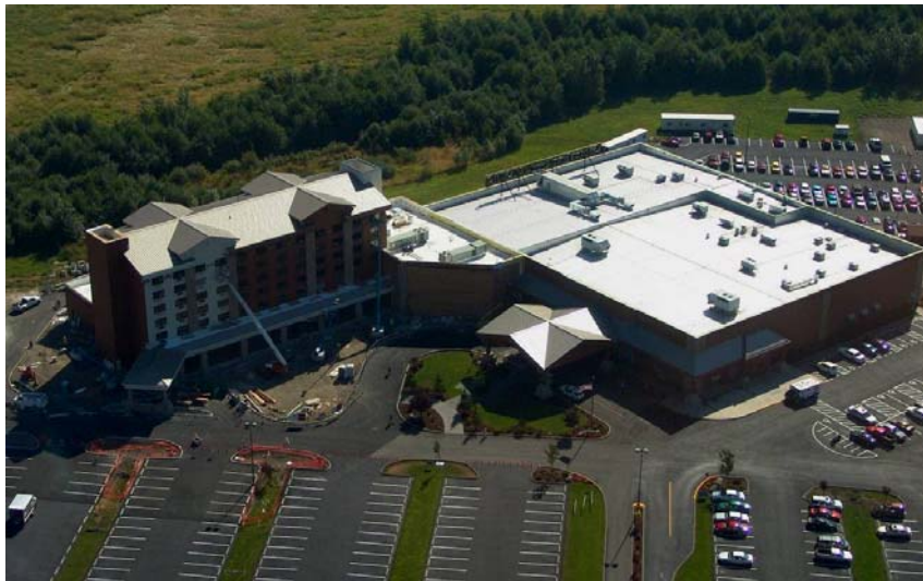
Figure 7-1 Aerial view of the finished Silver Reef Casino Hotel expansion (source, Hayward Baker, Inc.).
