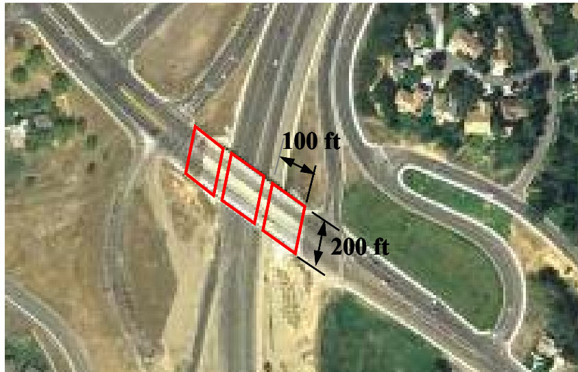
Figure 9-6 Aerial view of the three liquefaction mitigation treatment areas at the Cherry Hill Bridge case history.
