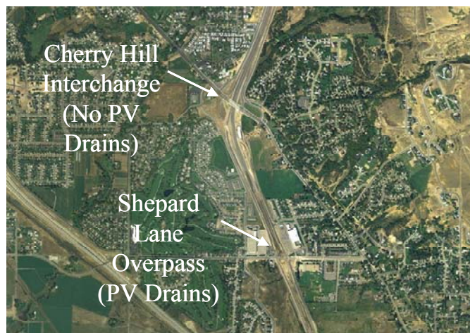
Figure 8-1 Aerial view of the Shepard Lane overpass which shows its proximity to the Cherry Hill interchange (within 1 mile). The Cherry Hill Bridge case history will be presented in Chapter 9.
