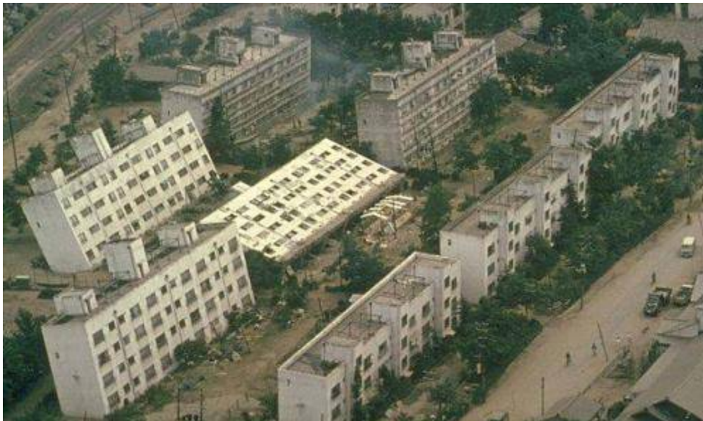
Figure 1-1 Settlement and tilting of apartment buildings in Niigata, Japan due to a M6.8 Earthquake in 1964 (source, Earthquake Engineering Research Center Library, University of California at Berkeley).
