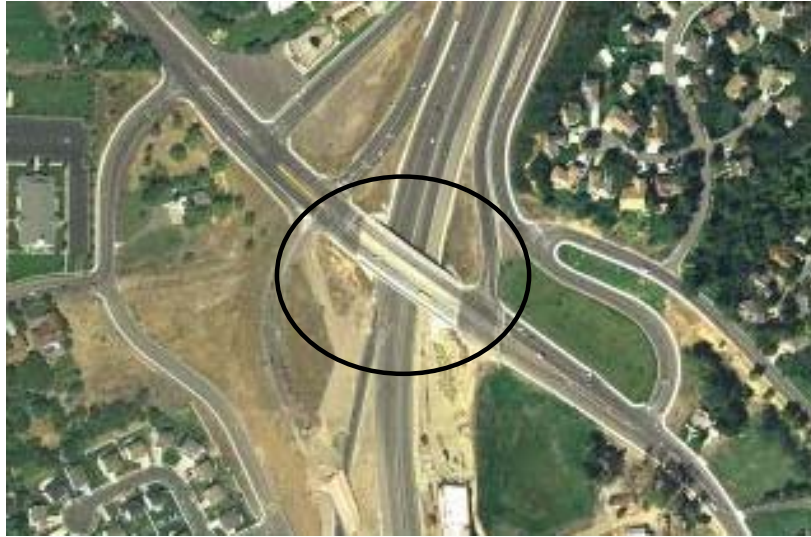
Figure 9-1 Aerial view of the Cherry Hill Bridge at the US 89 and Cherry Hill Interchange in Farmington, Utah.
