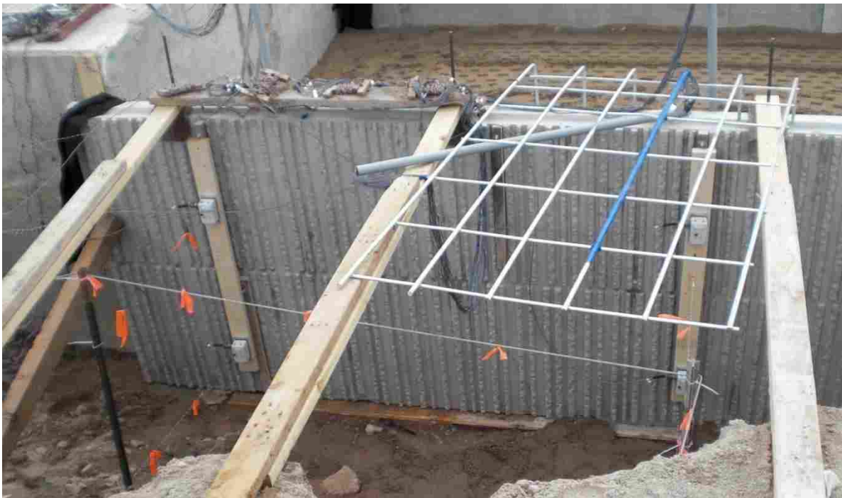
Figure 6.3: String Pot Configuration on MSE Panel for Loose Sand MSE Test
