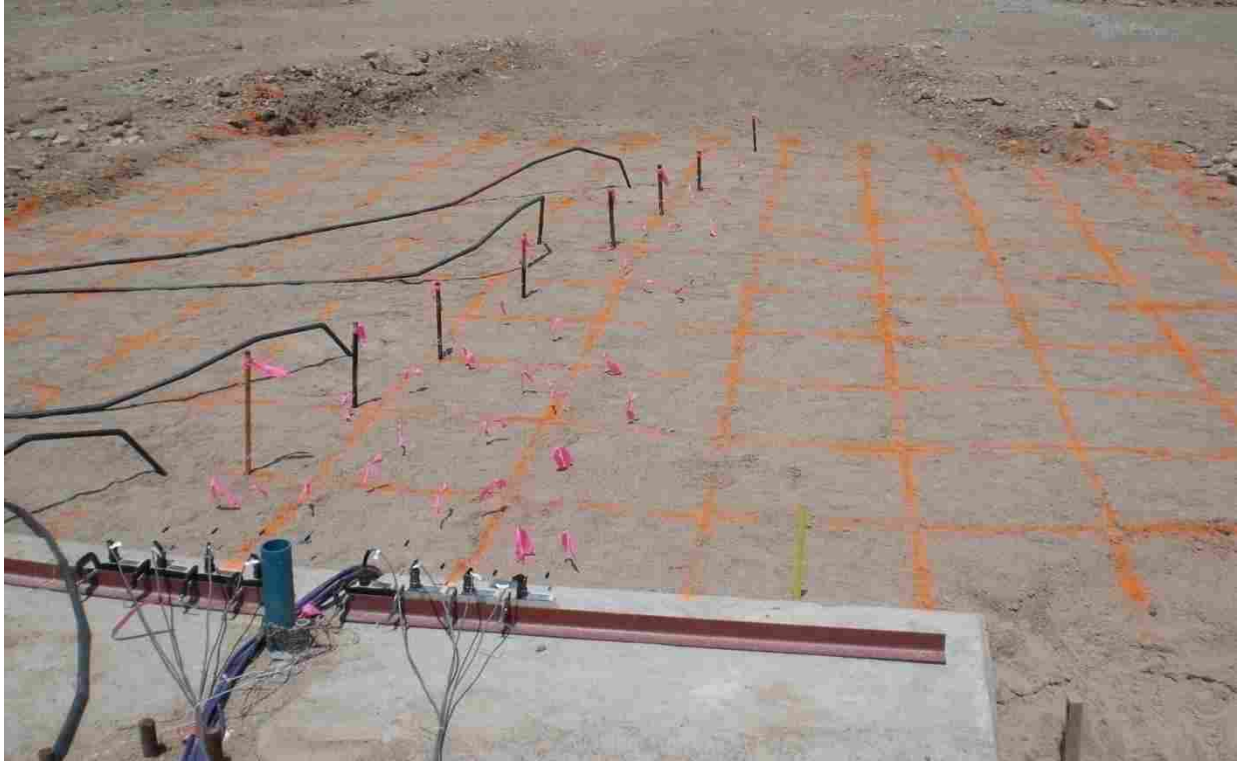
Figure 4.1: Photograph of the Loose Sand Unconfined (3D) Backfill Zone
