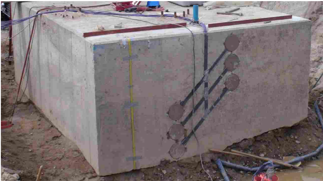
Figure 3.7: Photograph of Pressure Plates Embedded in the Pile Cap
