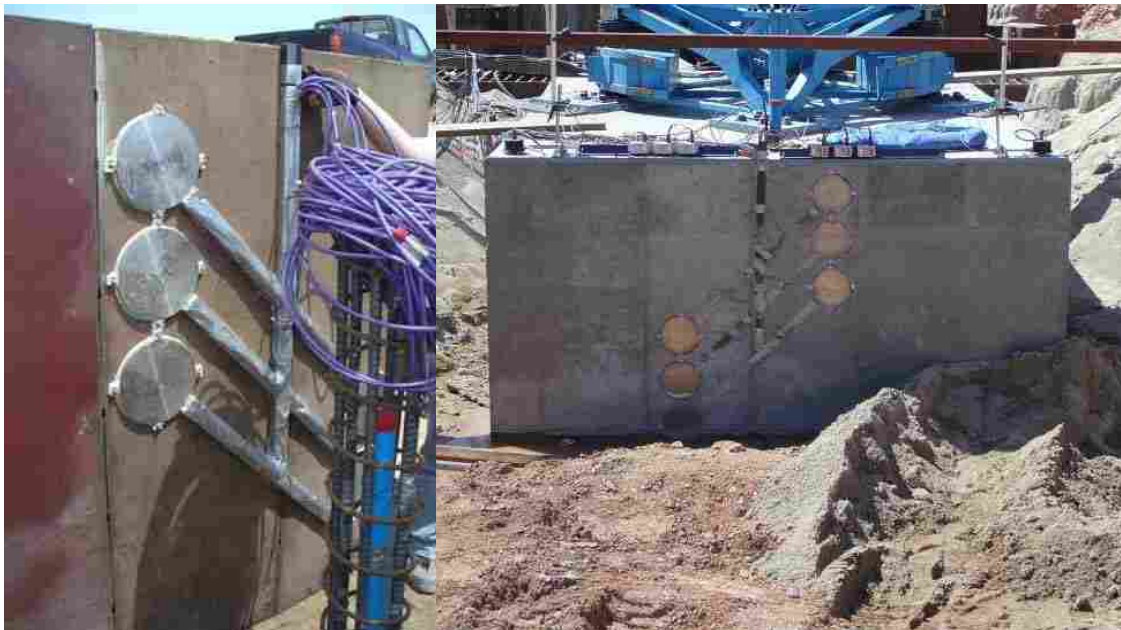
Figure 3-9 Pressure plates constructed on the north face of the pile cap
