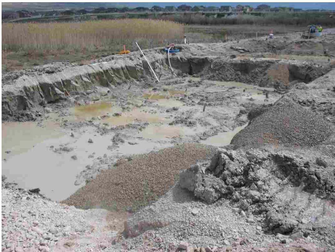
Figure 4-4. Excavation for Wall Embedment and Drainage Layer
