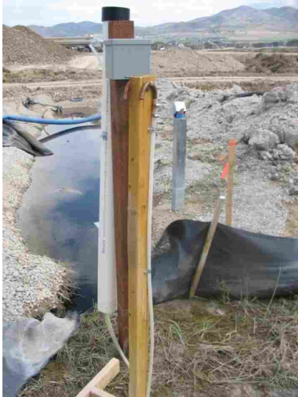
Figure 3-5. Manometer Settlement Platform
