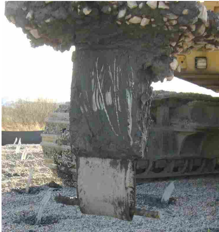
Figure 3-10. Mandrel with PV Drain and Rebar Anchor Prior to Installation
