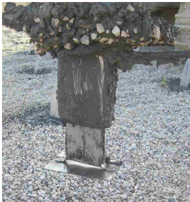
Figure 3-11. Mandrel with PV Drain and Plate Anchor Prior to Installation
