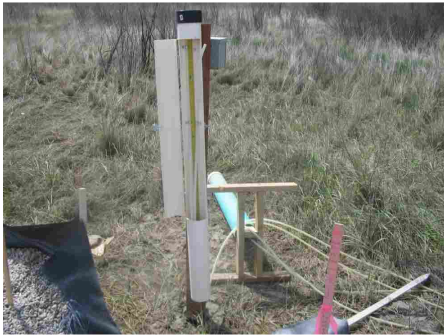
Figure 3-6. Manometer Gauge Box
