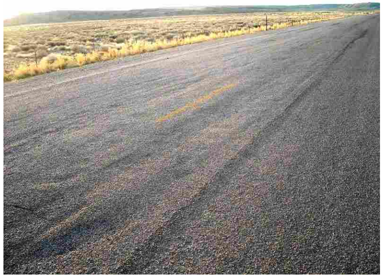
Figure 4.5 Rutting distress.
