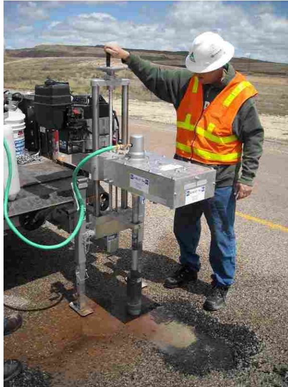
Figure 3.12 Truck-mounted coring rig.
