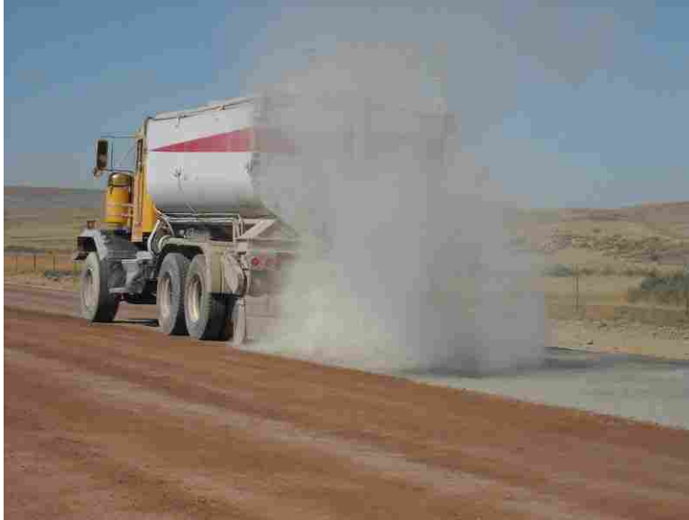
Figure 3.2 Distribution of the cement with a cement spreader truck.
