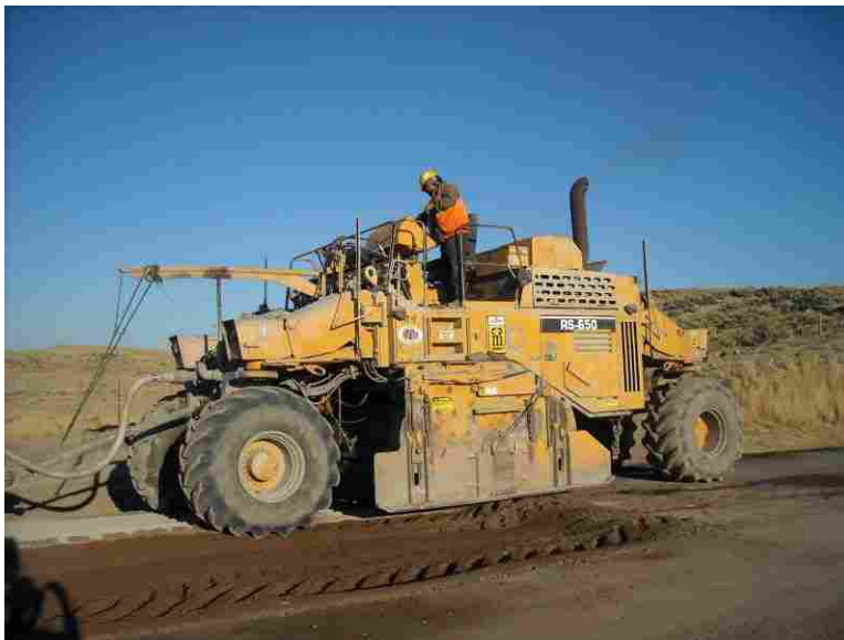
Figure 3.3 In-situ mixing of the base, RAP, and cement with a reclaimer.
