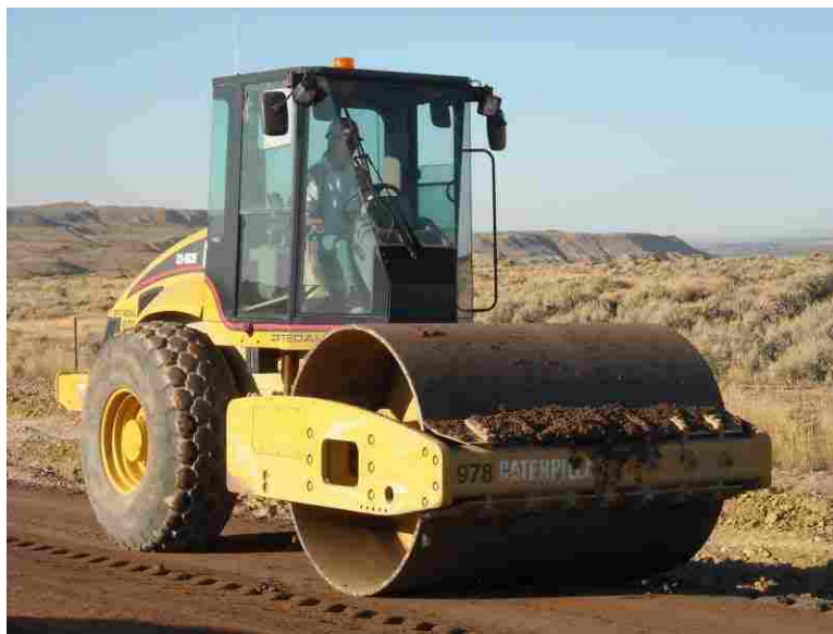
Figure 3.4 Compaction with a vibratory roller.
