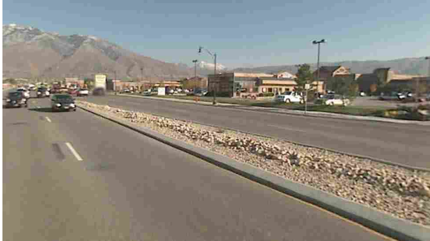
Figure 3-4. Raised median on 12300 South (SR 71) (Google 2010).
