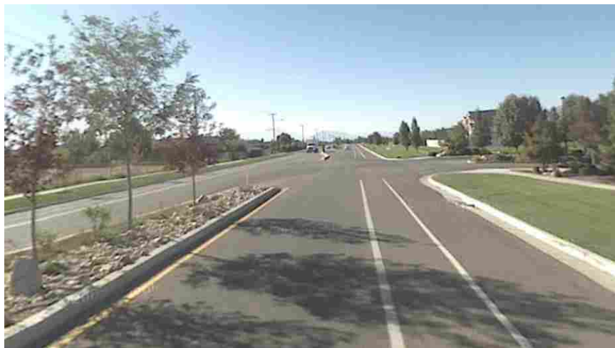
Figure 3-2. Raised median on Alpine Highway (SR 74) (Google 2010).
