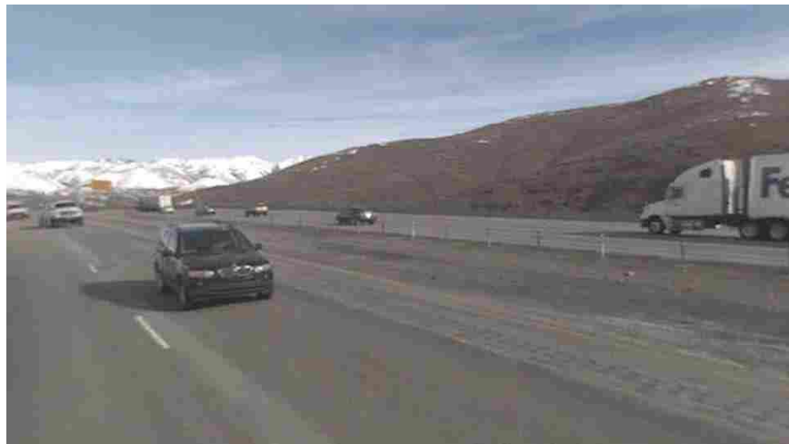
Figure 3-14. I-80 near Lamb's Canyon Interchange.
