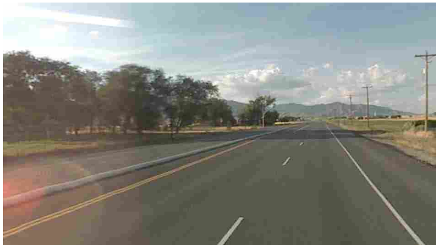
Figure 3-6. Raised median on SR 36 (Google 2010).
