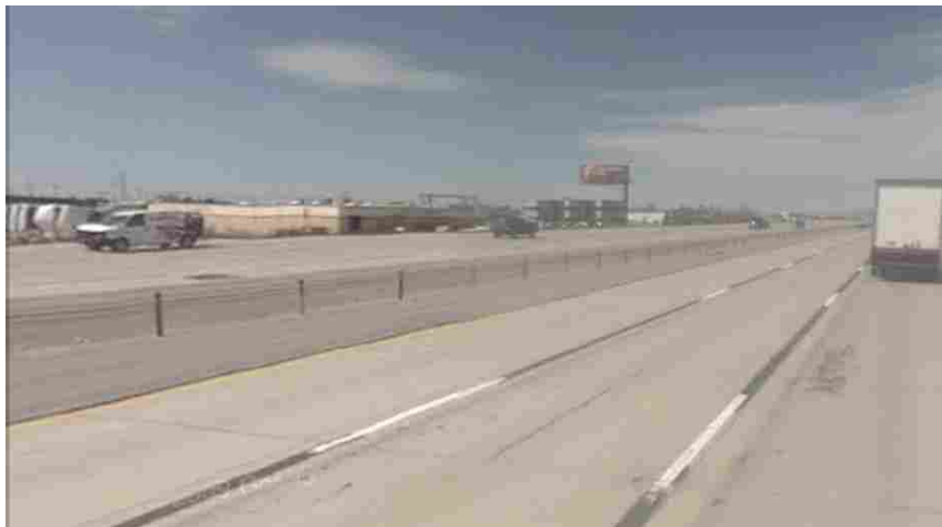
Figure 3-13. I-215 West between 2100 South and 4500 South in Salt Lake (Google 2010).
