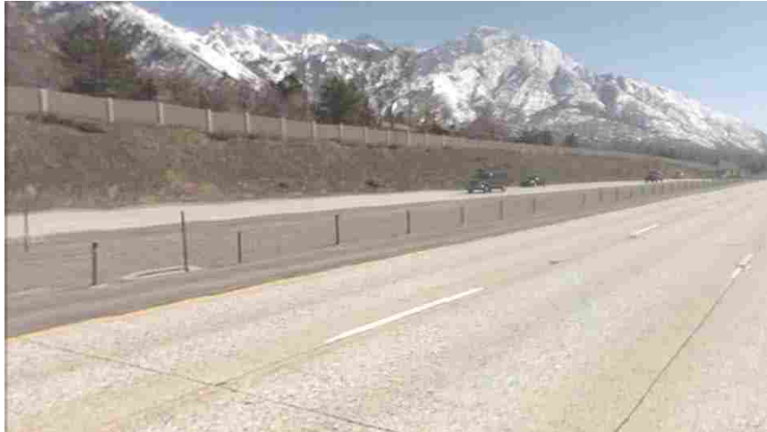
Figure 3-12. I-215 East between 3100 South and 3800 South in Salt Lake (Google 2010).
