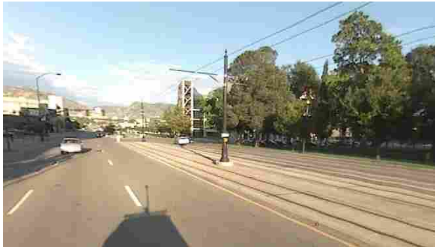
Figure 3-3. Raised median on 400/500 South (SR 186) (Google 2010).
