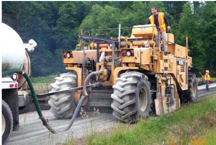
Figure 2.7 Mixing cement with road base while injecting water (Luhr et al. 2005).
