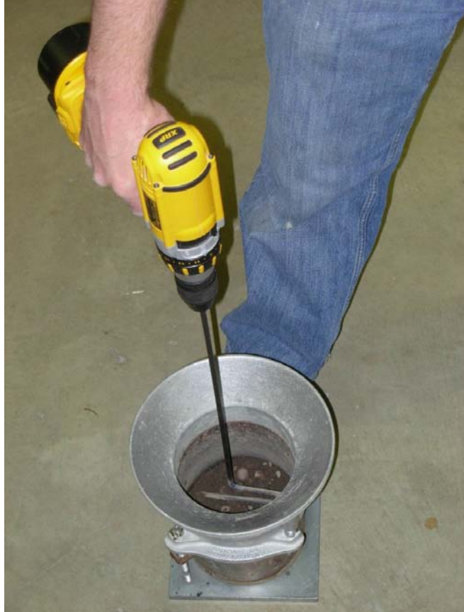
Figure 3.15 Mixing cement with aggregate.
