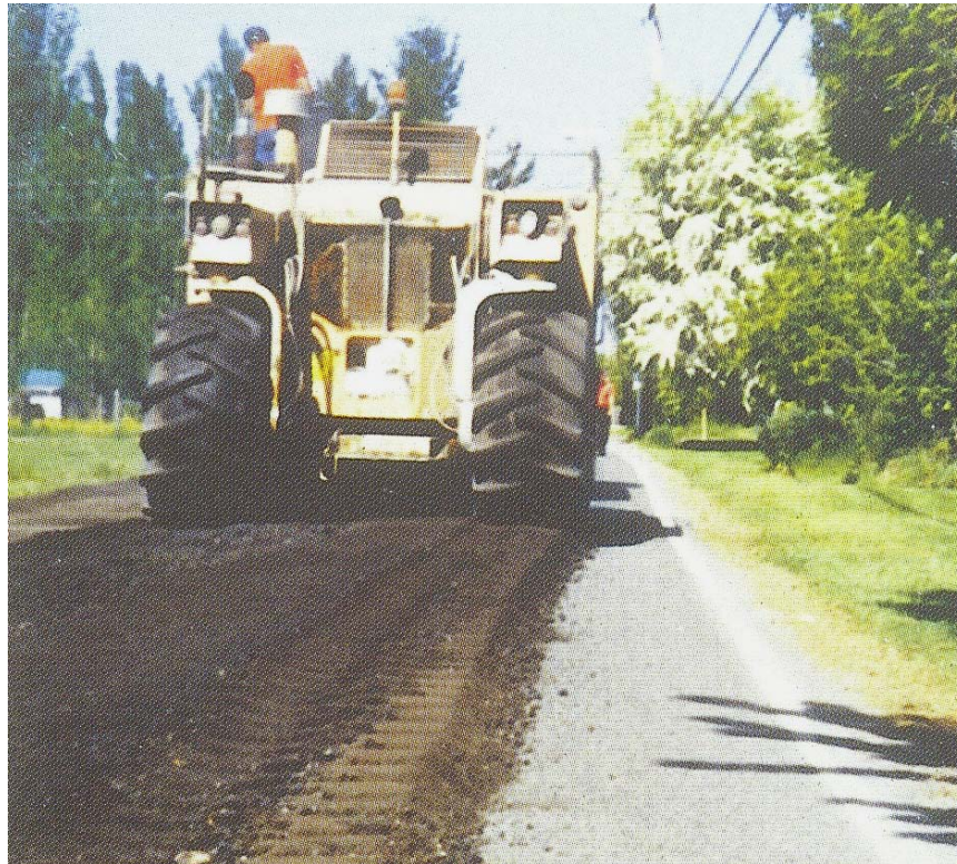
Figure 2.2 Grinding a failed asphalt pavement and mixing with underlying road base (PCA 2002).
