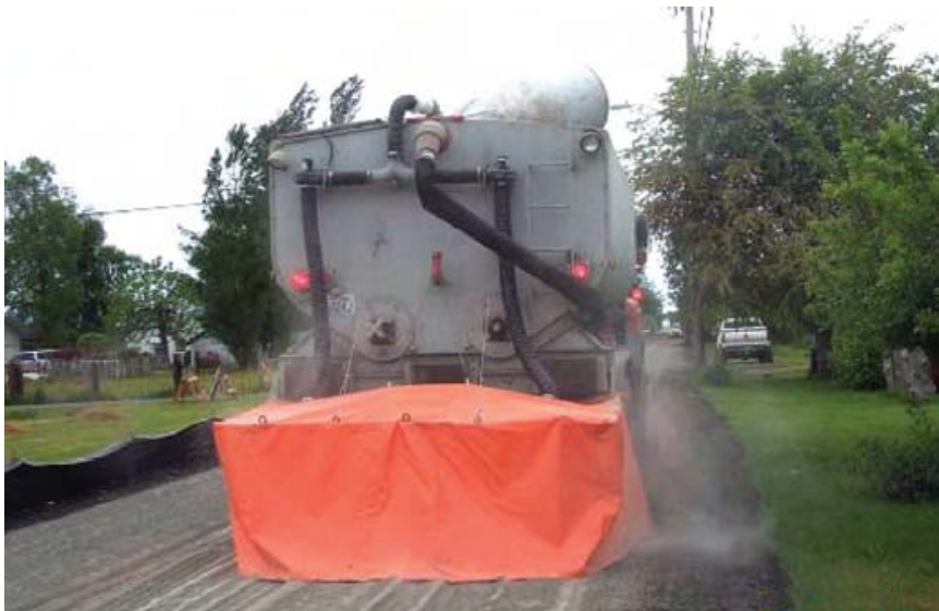
Figure 2.4 Spreading dry cement using a pneumatic spreader with an enclosure for dust reduction (Luhr et al. 2005).
