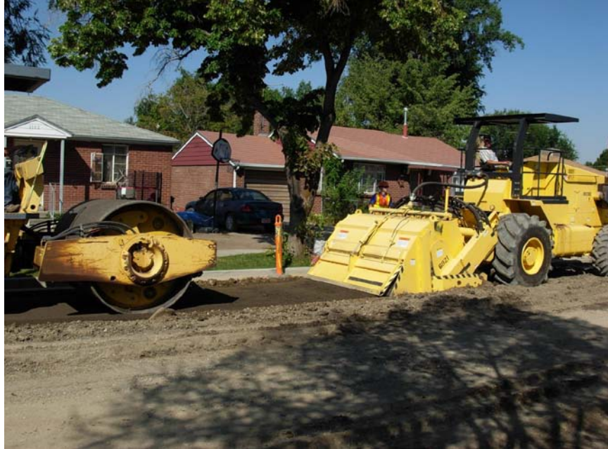
Figure 2.8 Compaction following mixing of cement and road base.
