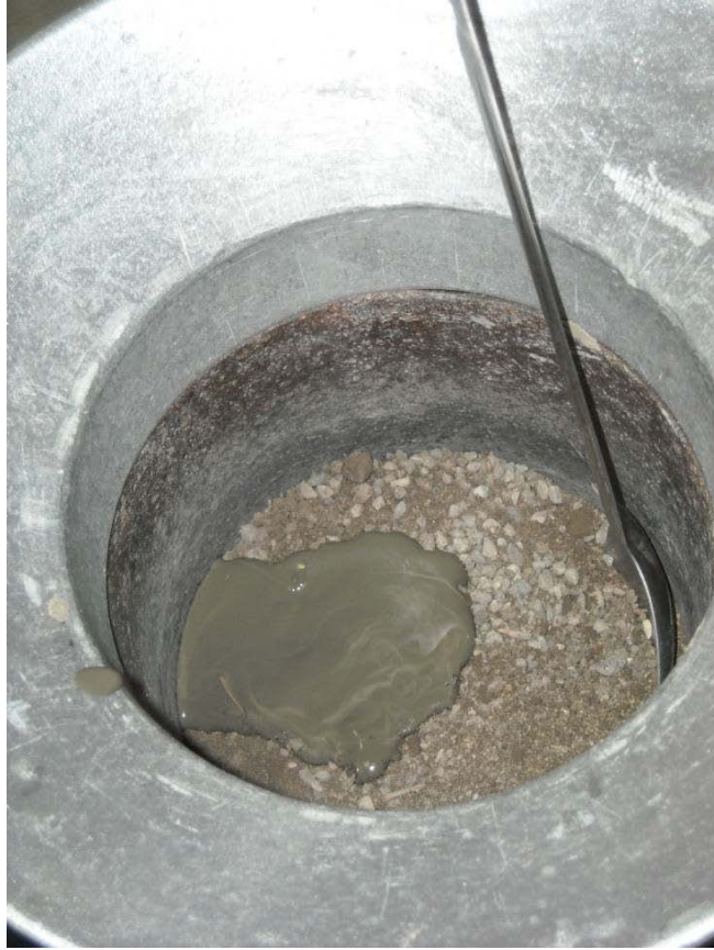
Figure 3.14 Cement slurry with aggregate before mixing.
