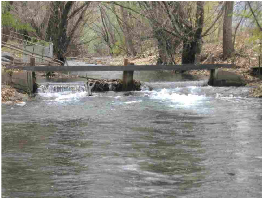
Figure A-1. Temporary diversion separating Reaches 1 and 2.
