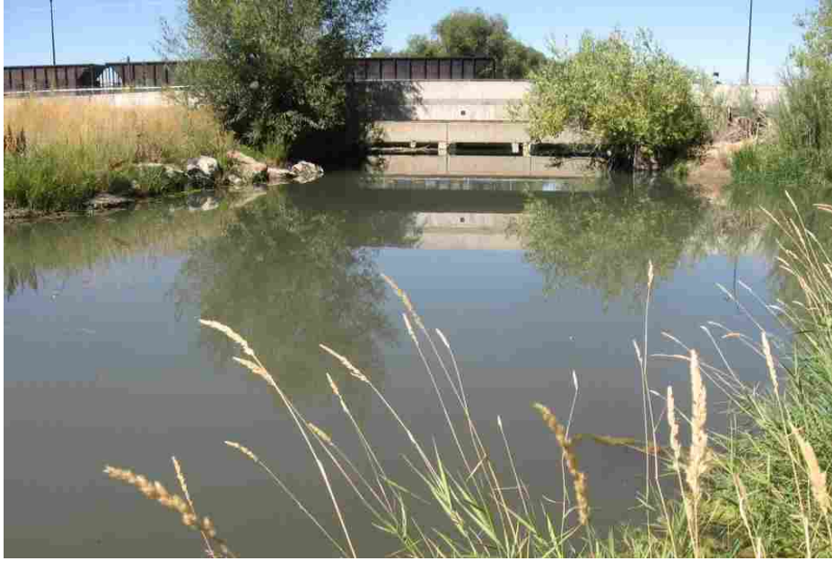
Figure A-2. Looking downstream at 1650 W crossing with backwater section.
