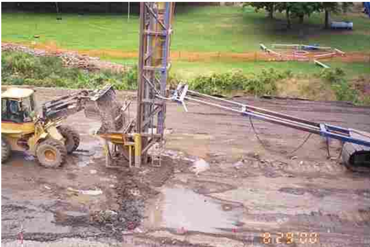
Figure 2.6 Water escaping through previously installed wick drains during stone column installation.
