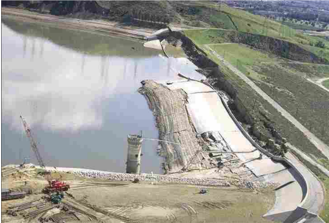
Figure 1.1 Destruction caused by liquefaction at the Van Norman Dam following the San Fernando Earthquake (source, www.ce.washington.edu ).
