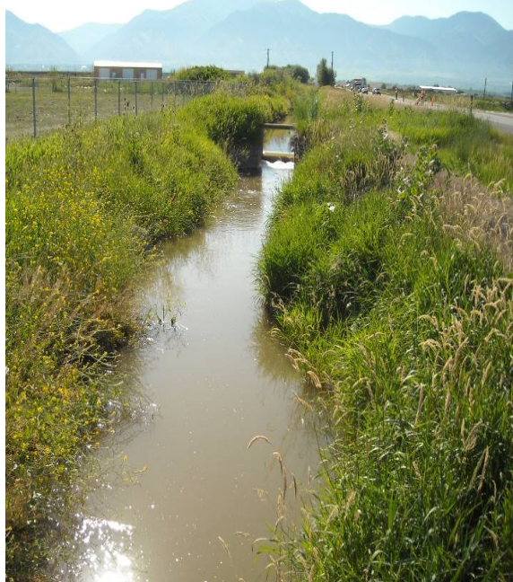
Figure 3.2 Irrigation Canal along Westbound State Route 30
