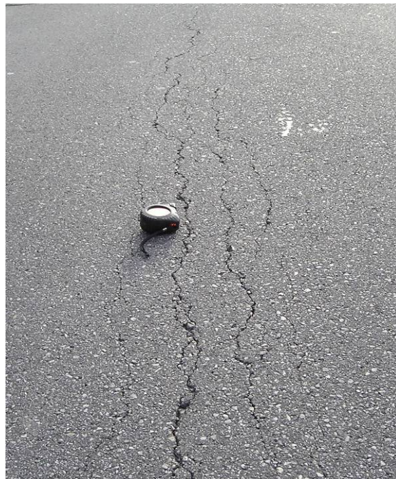
Figure 2.4 Fatigue Cracking
