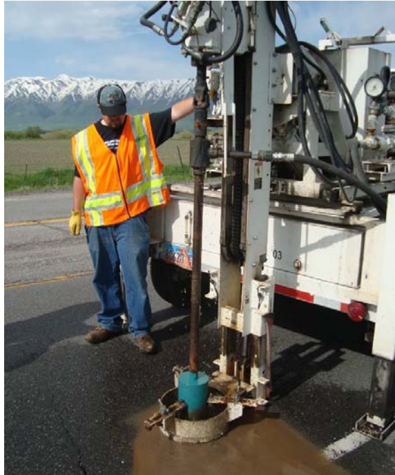
Figure 3.9 Coring of Asphalt Layer
