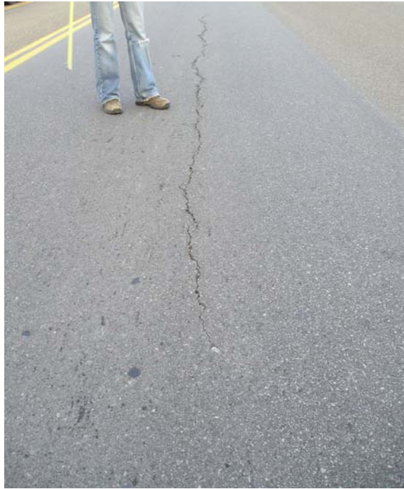
Figure 2.2 Longitudinal Cracking
