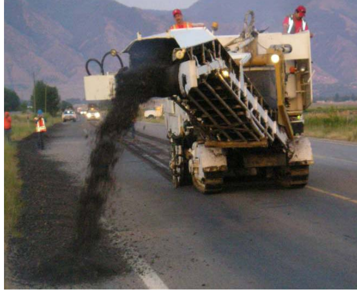
Figure 3.3 Milling of Existing Asphalt Surface
