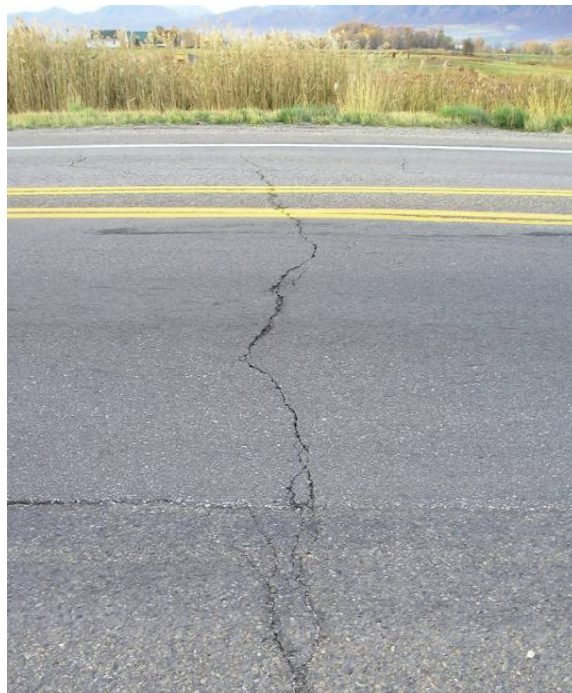
Figure 2.3 Transverse Cracking
