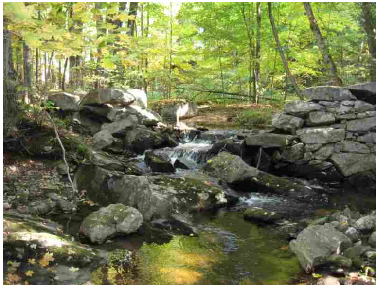
Figure 3-15: Possible fish barrier downstream of Falmouth culvert. The presence of this very old retention structure allowed for experimental retrofit.
