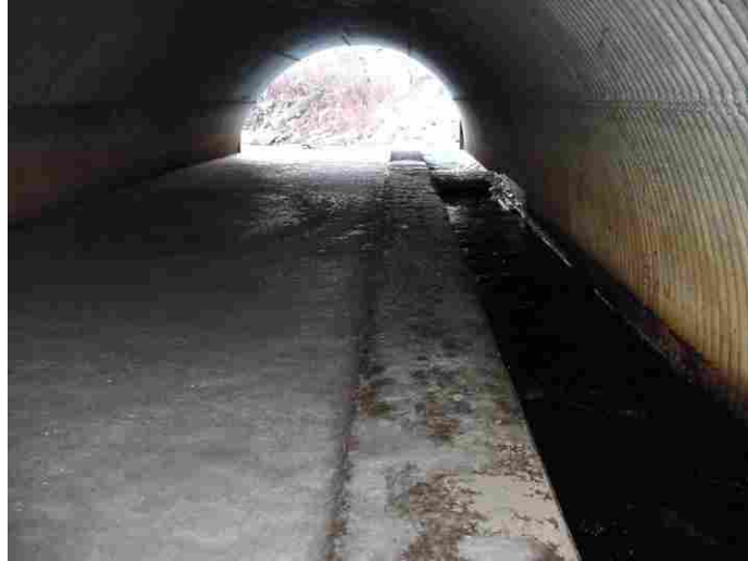
Figure 2-15: Looking towards culvert outlet. Longitudinal channel on right. (CALTRANS 2007)
