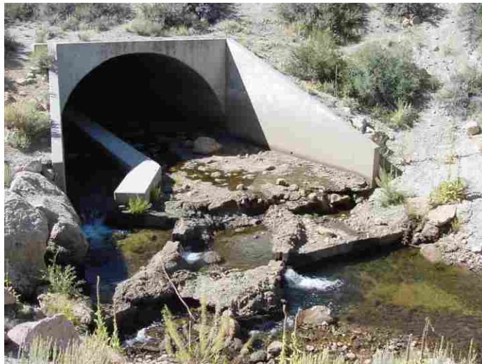
Figure 2-16: Looking at culvert outlet. Longitudinal Channel on left. (CALTRANS 2007)
