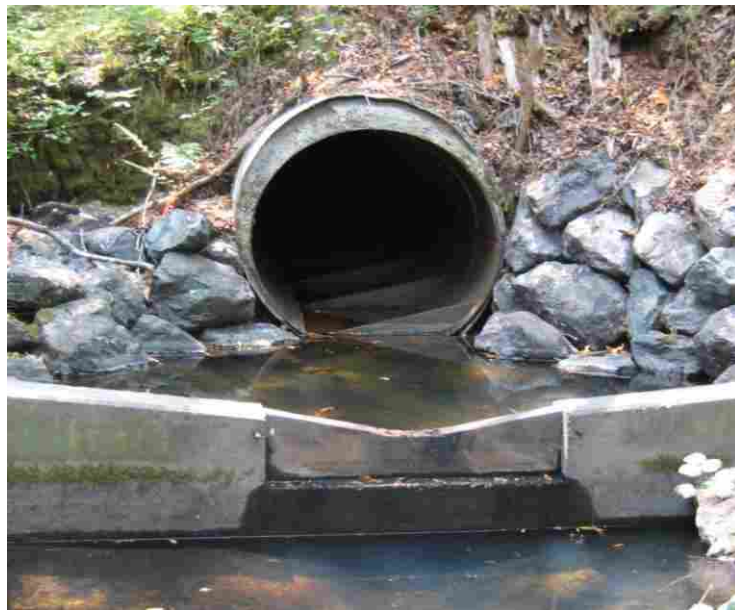
Figure 3-6: Outlet of slip lined culvert retrofit of John Hatt Creek showing corner baffles and one of the three tailwater control barriers.
