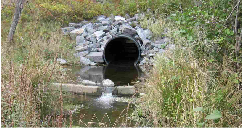
Figure 3-8: Culvert retrofit outside Belfast, Maine, showing tailwater control weir.
