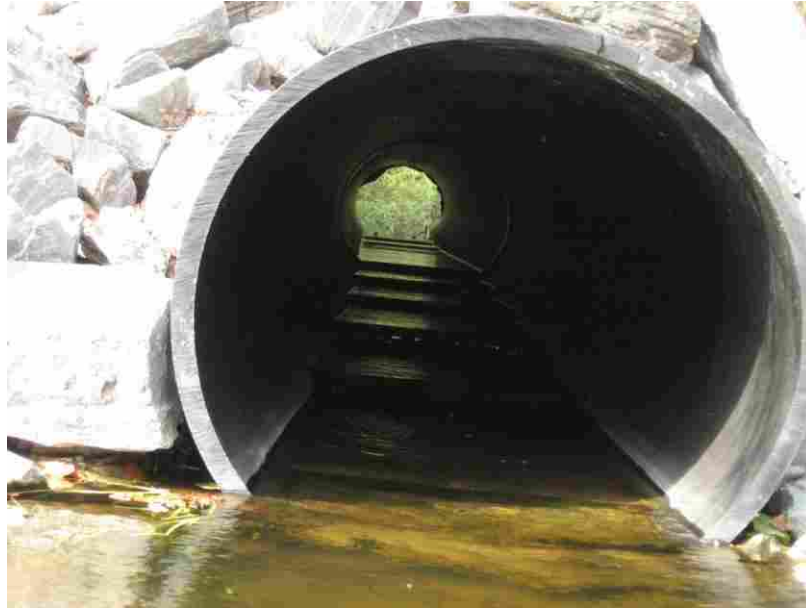
Figure 3-10: View of all baffles within Belfast, Maine culvert retrofit.
