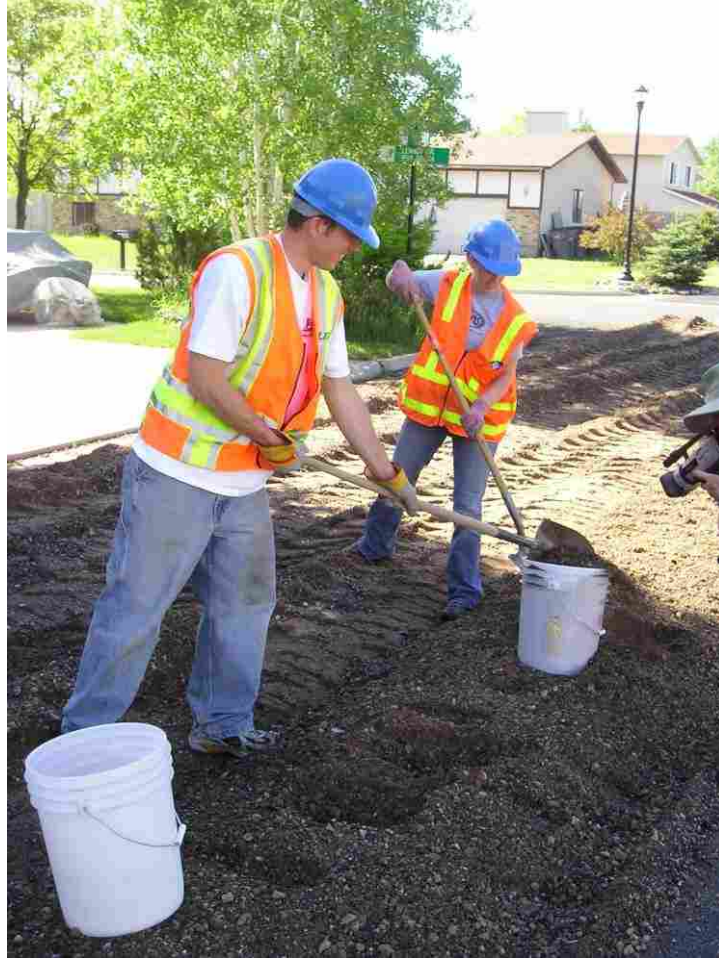
FIGURE 3.9 Material sampling just after reclamation.
