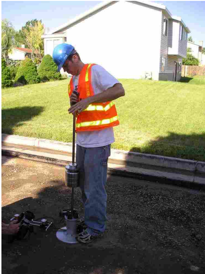
FIGURE 3.10 PFWD testing just after reclamation.
