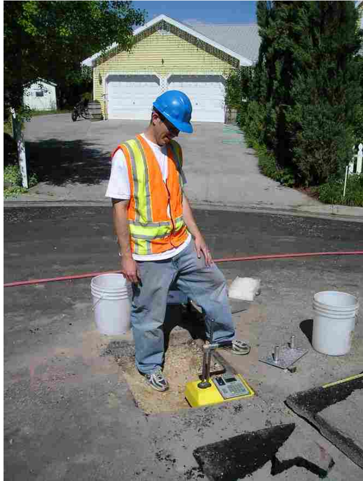
FIGURE 3.7 NDG testing just before reclamation.
