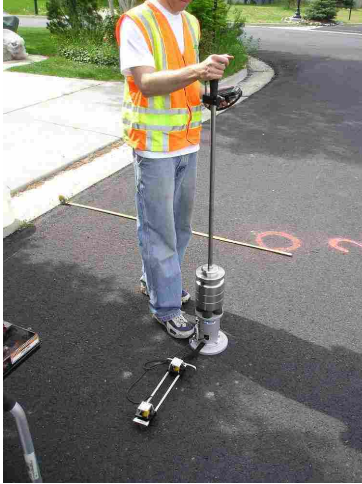
FIGURE 3.5 PFWD testing just before reclamation.
