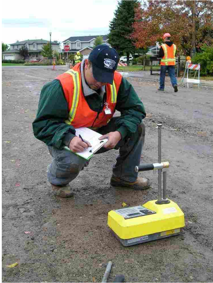
FIGURE 3.12 NDG testing just after reclamation.
