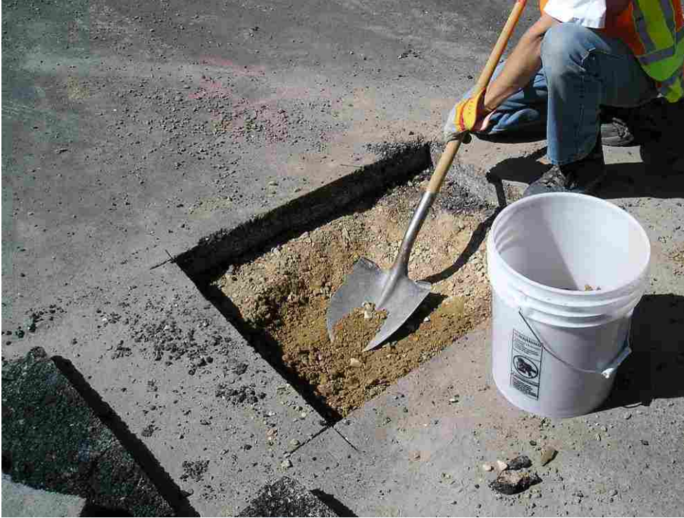
FIGURE 3.8 Material sampling just before reclamation.
