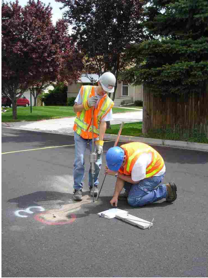
FIGURE 3.6 DCP testing just before reclamation.
