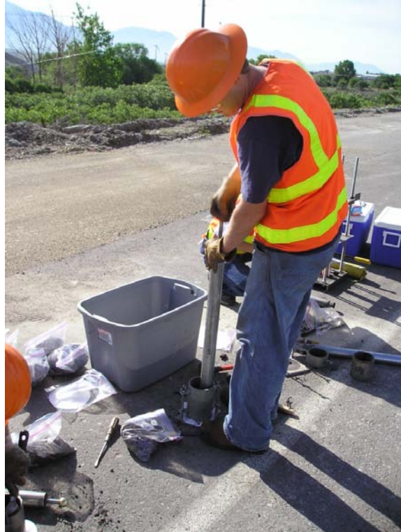
Figure 3-10: Manual compaction.
