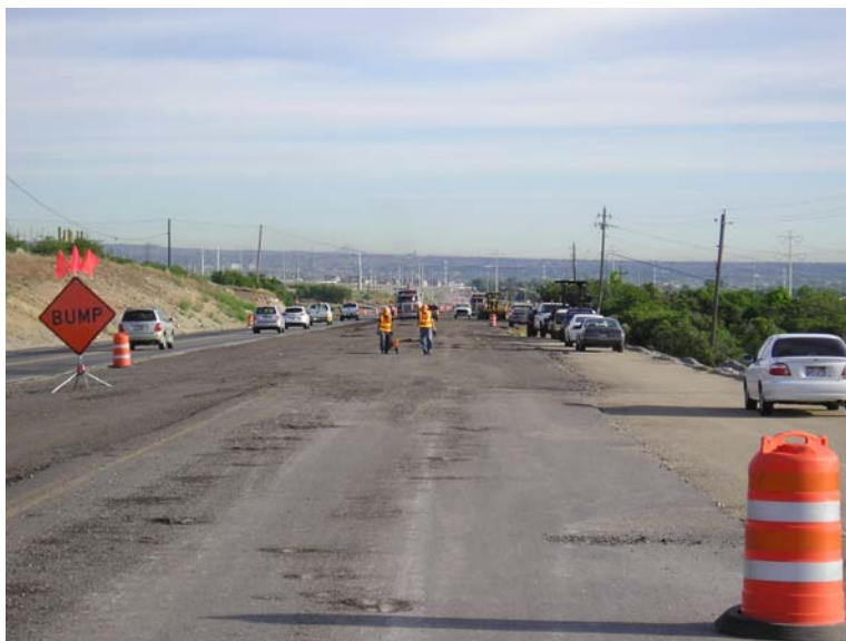
Figure 3-2: Redwood Road during reconstruction.
