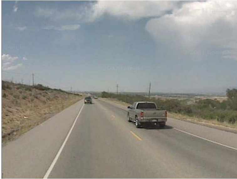
Figure 3-1: Redwood Road before reconstruction.
