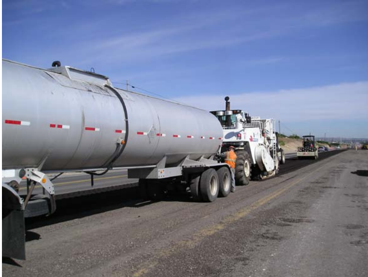
Figure 2-1: Injection of emulsion.
