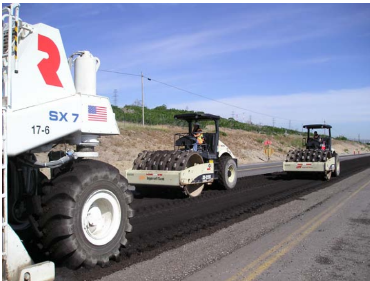
Figure 2-2: Compaction of emulsion-treated base.
