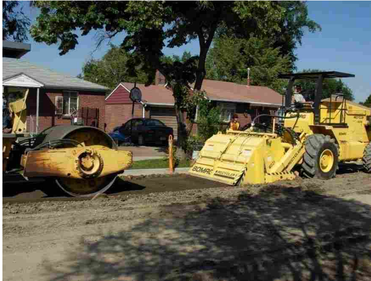
Figure 3-10: Mixing and compacting CTB layer.
