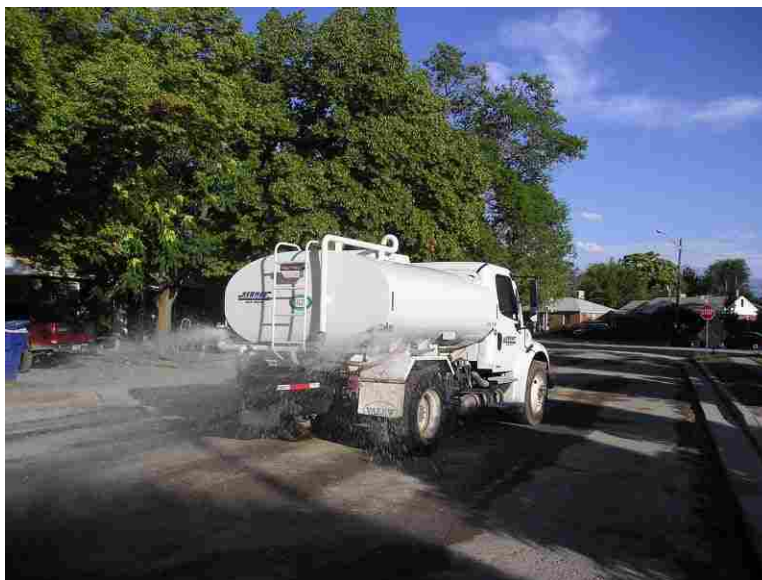
Figure 2-5: Moist curing using a water truck.
