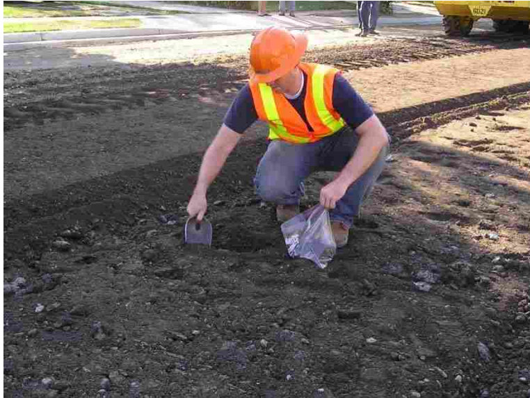
Figure 3-7: Sampling of RAP-base blend.
