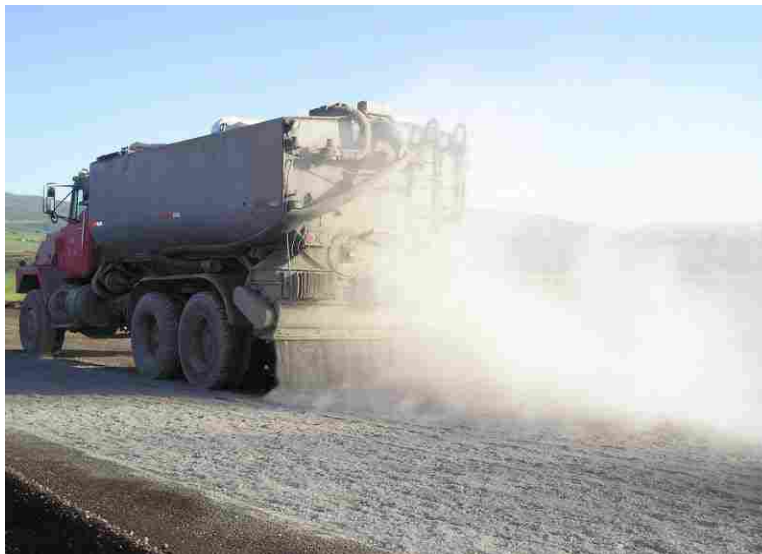
Figure 2-1: Cement powder application.
