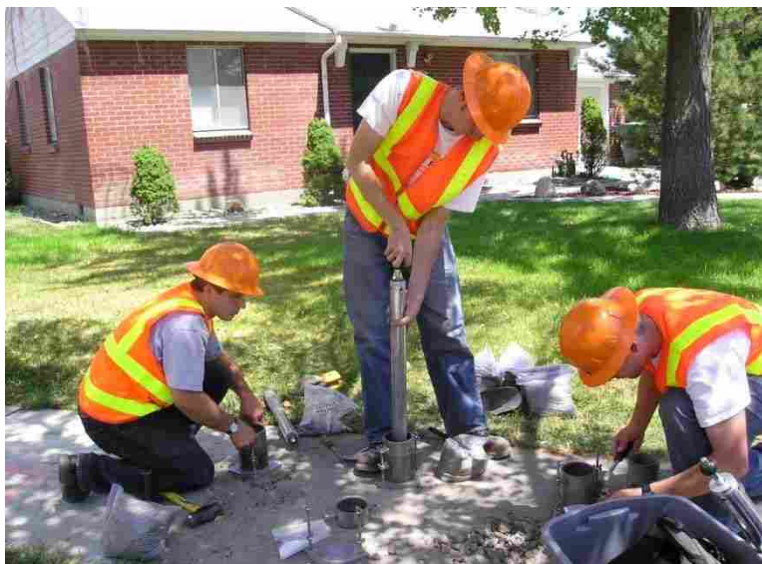
Figure 3-9: Compacting field specimens.
