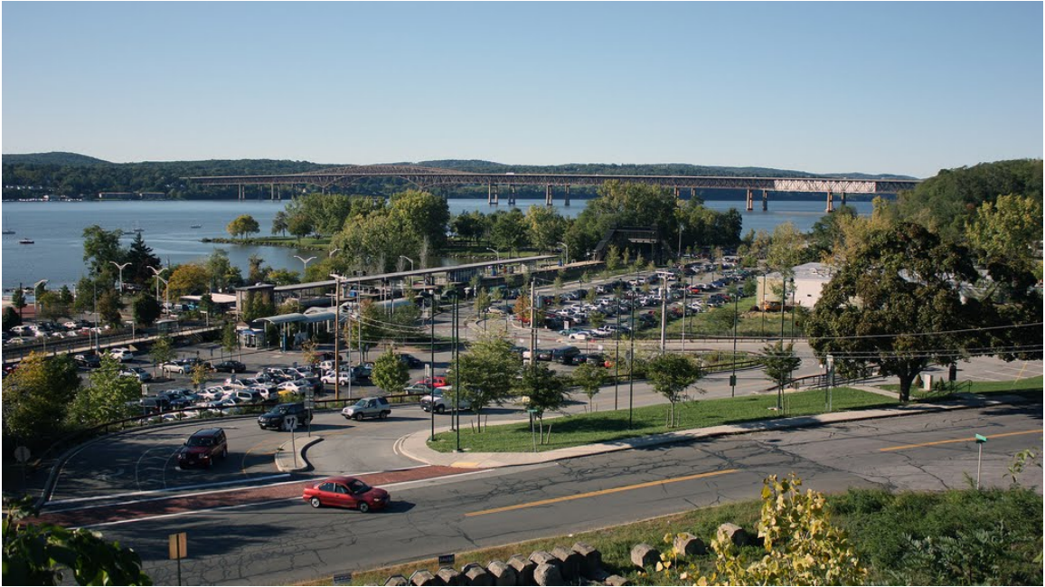
Figure 17 - Existing Beacon Station From < http://www.panoramio.com/photo/41603054 >
