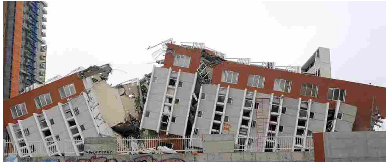
Figure 1.1: A building in Concepcion, Chile after the 2010 earthquake. The condition of the building would expose rescuers to a great amount of risk. The condition also offers a tremendous challenge in exploration. The walls could not be used as assumed structure for navigation (since they are no longer vertical), and the slanted floors would exclude a ground robot.
