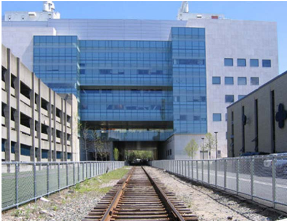
Figure 15 - Bridge over the Rail Way (Haley & Aldrich, Inc. 2008)
