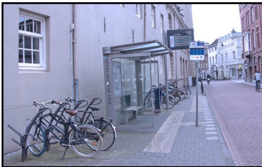
Fig. 1. The Bicycle Master Plan looked at a wide variety of cycling related issues, including how to improve bicycle parking at bus stops. Photo by the author.
