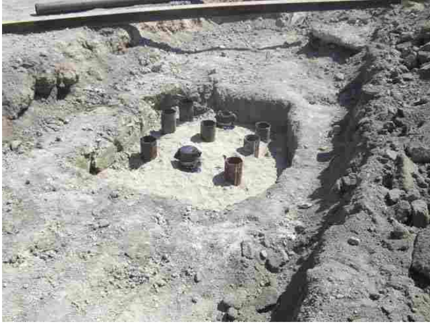
Figure 4-2 - Driven pile layout prior to cap construction.
