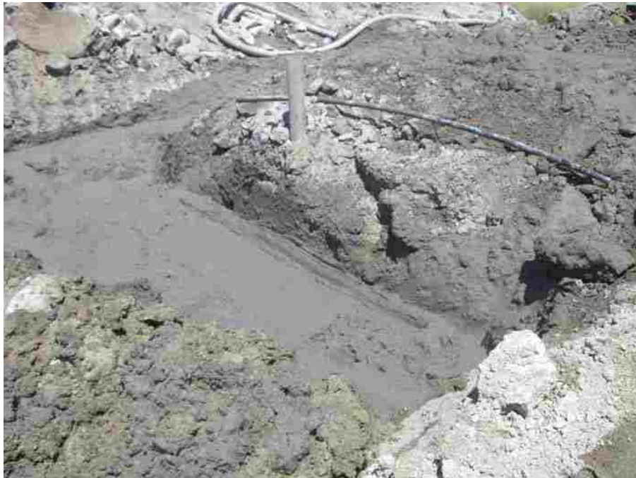
Figure 4-13 – Photograph of the finished mass mixed zone.
