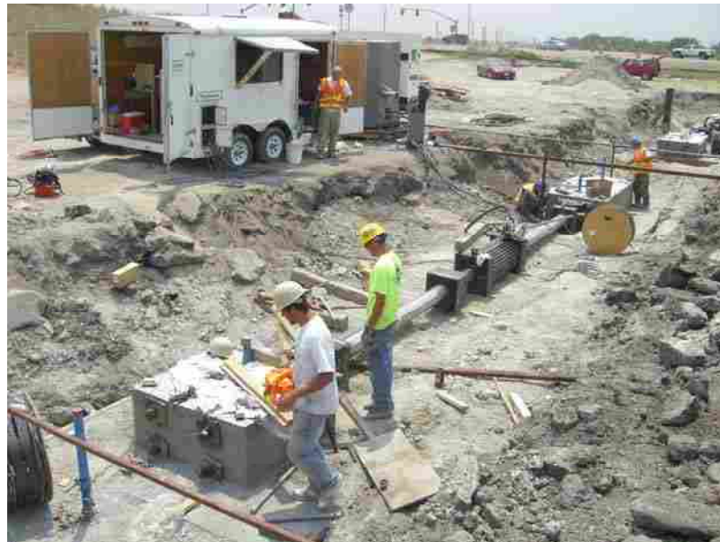
Figure 4-10 - Photo of actuator setup between caps 1 & 2.
