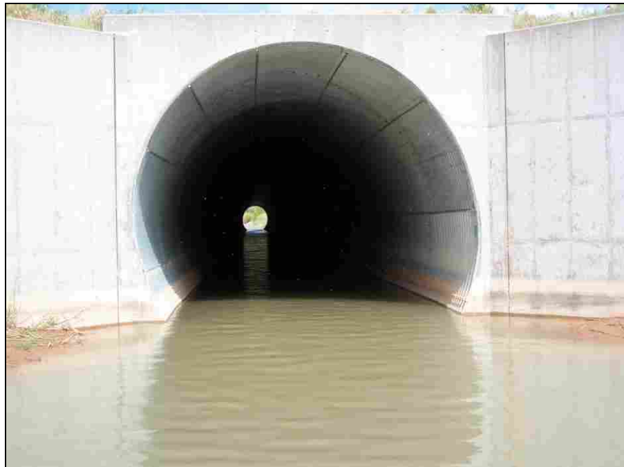
Figure 4-11: Outlet of Backwatered Culvert #2
