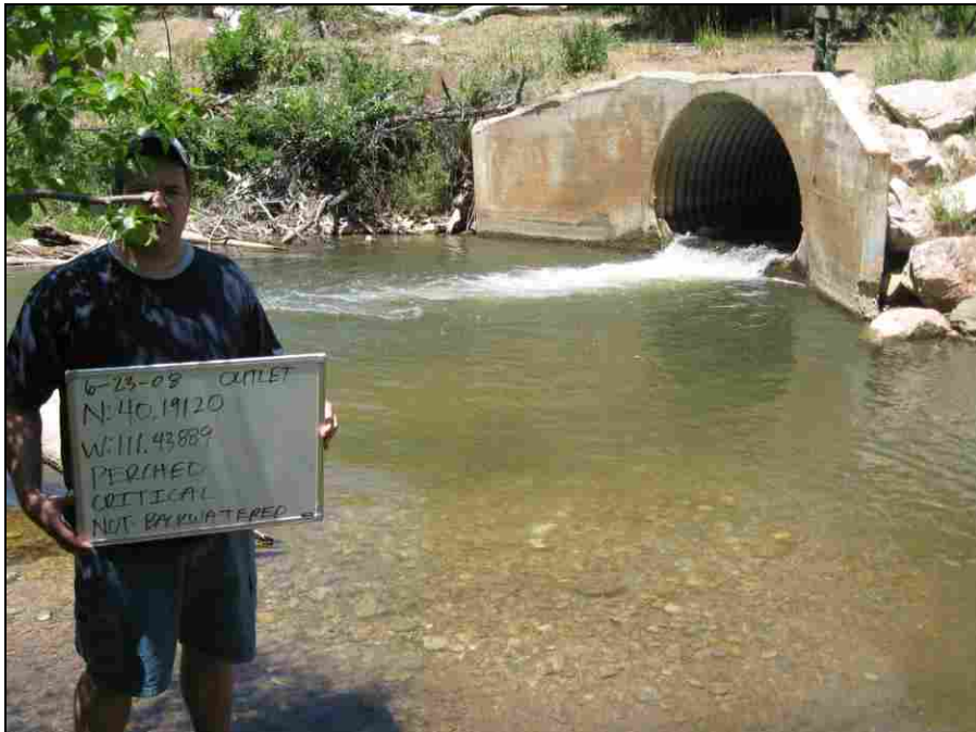
Figure 4-4: Hydraulic Evaluation Photo Taken at the Outlet
