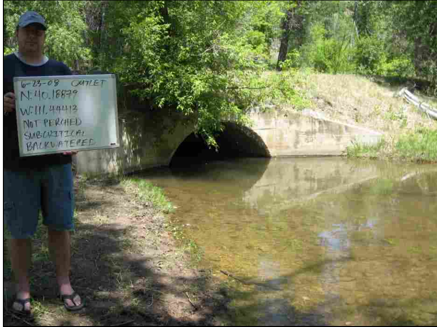
Figure 3-3: Hydraulic Evaluation Photo of a Culvert Outlet
