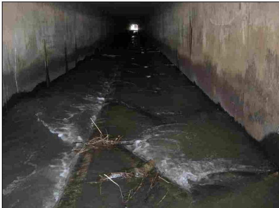
Figure 5-12: Photo of Fish Baffles Mid-Culvert
