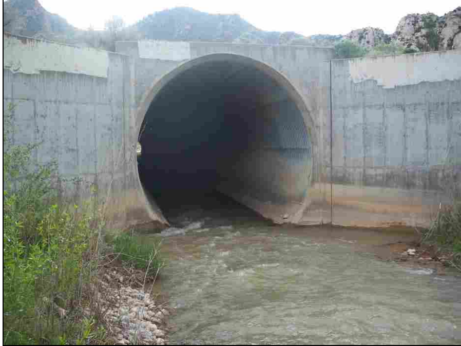
Figure 6-10: Soldier Creek Culvert Inlet (Soldier Creek Field Verification Site)
