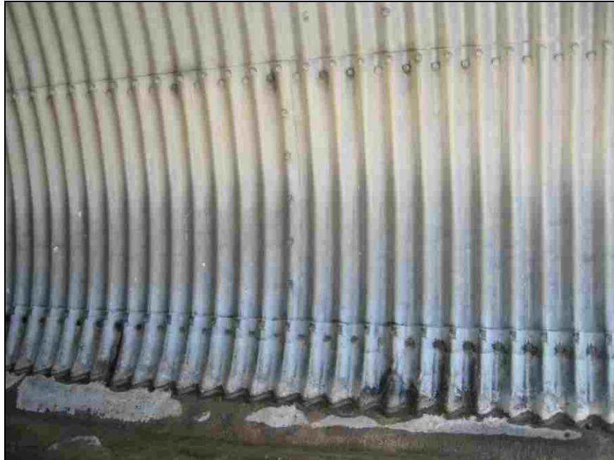
Figure 5-34: Plated Culvert
