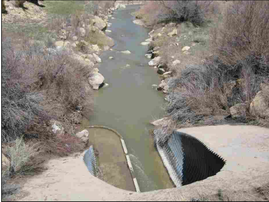
Figure 5-1: Embankment Looking Upstream Photo
