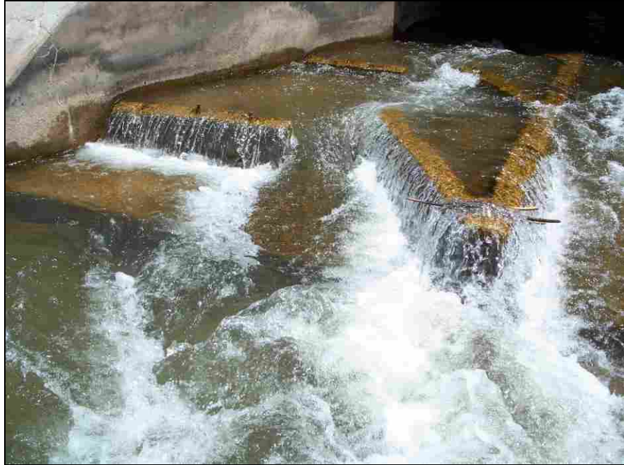
Figure 5-11: Photo at Outlet of Fish Baffles
