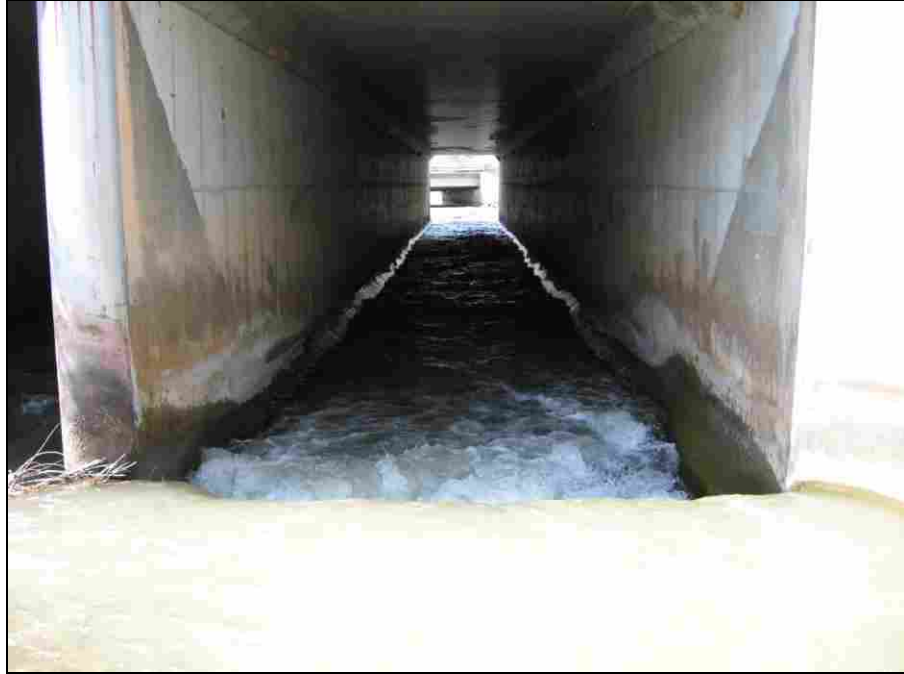
Figure 5-15: Spillway at Inlet
