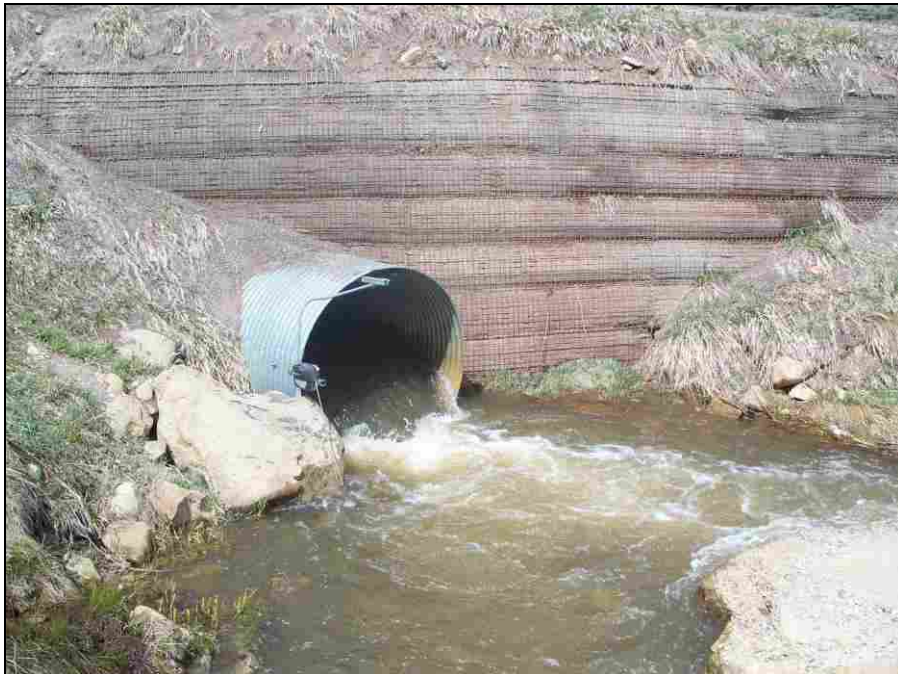
Figure 5-23: Gabion Wall
