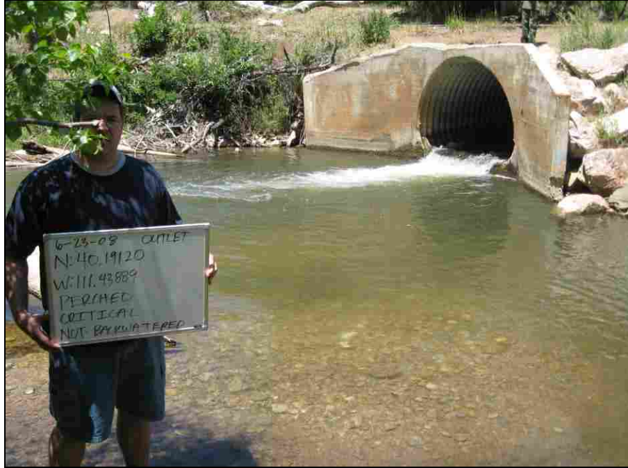
Figure 3-5: Hydraulic Evaluation Photo of a Culvert Outlet
