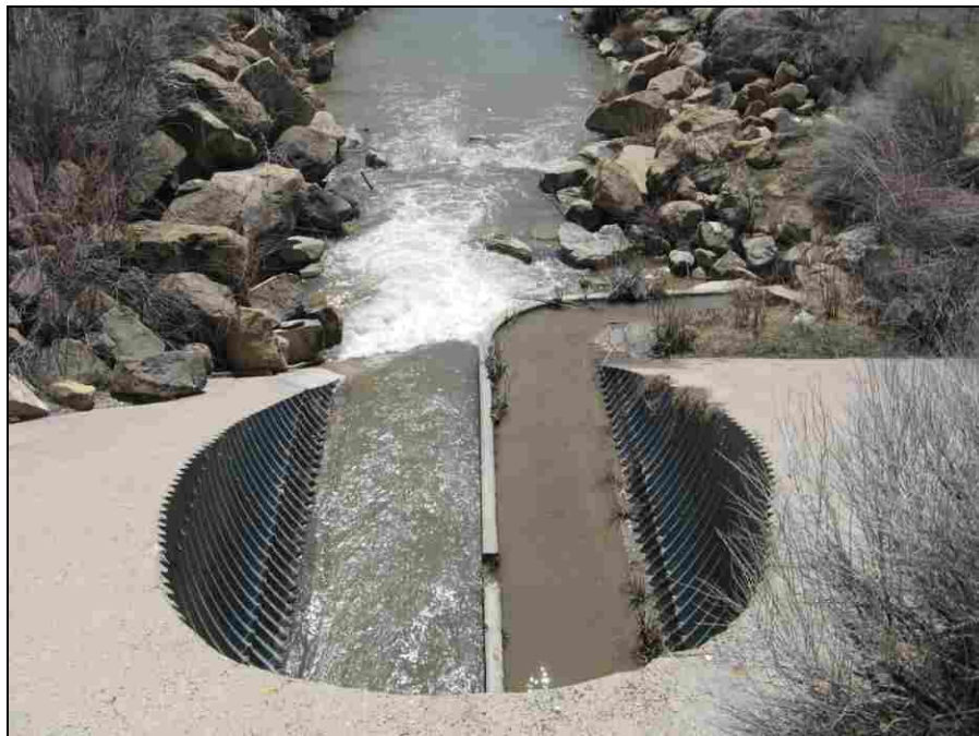
Figure 6-23: Salina Creek Culvert Outlet and Wildlife Trail Looking Downstream
