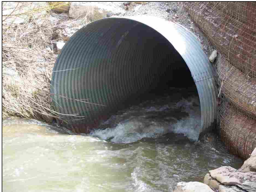
Figure 5-43: Hydraulic Jump Just Inside Culvert Inlet
