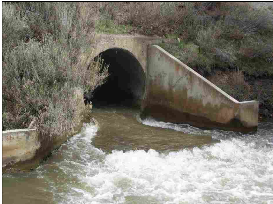
Figure 5-45: Hydraulic Jump at End of Outlet Apron
