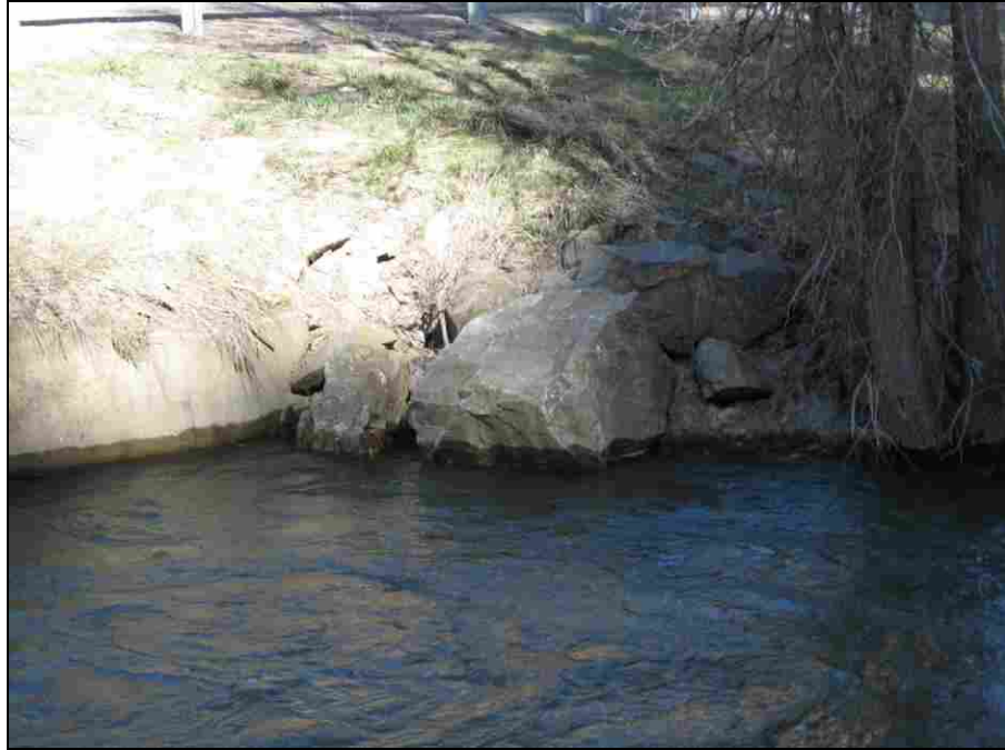
Figure 5-21: Riprap at Toe of Outlet Wingwall
