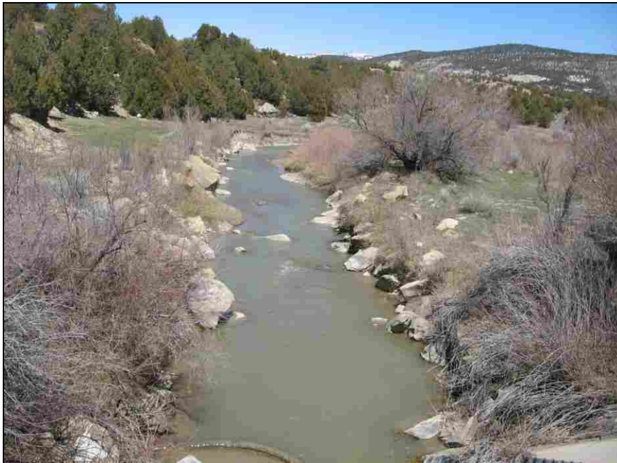
Figure 5-2: Additional Embankment Looking Upstream Photo Showing Floodplain
