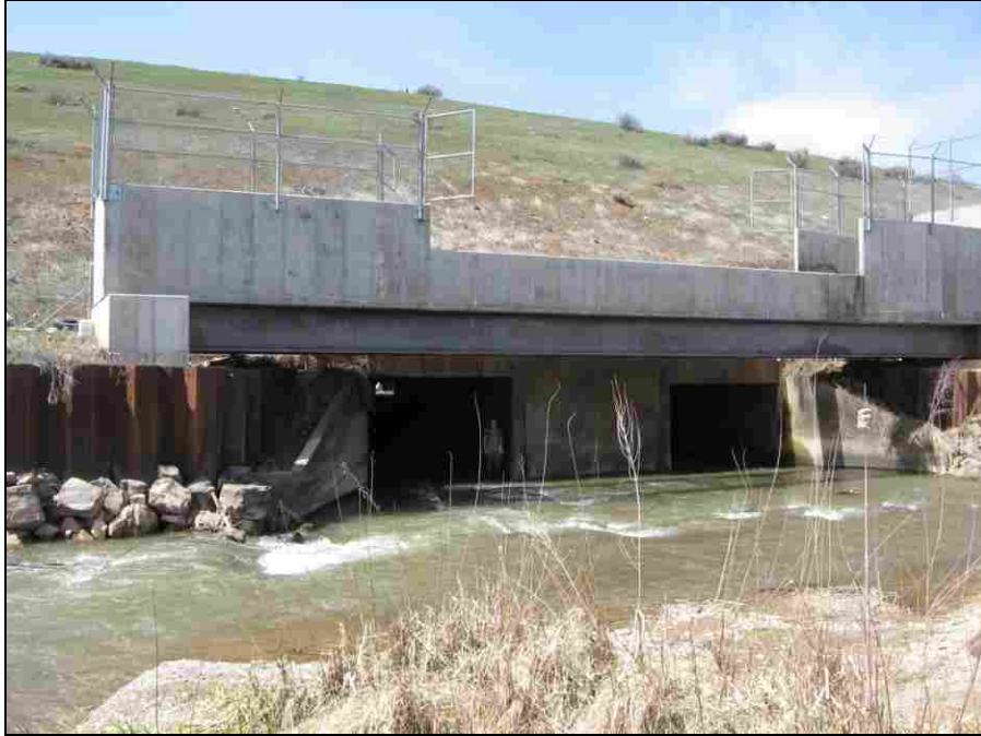
Figure 6-6: Diamond Fork Culvert #2 Inlet (Diamond Fork Field Verification Site)
