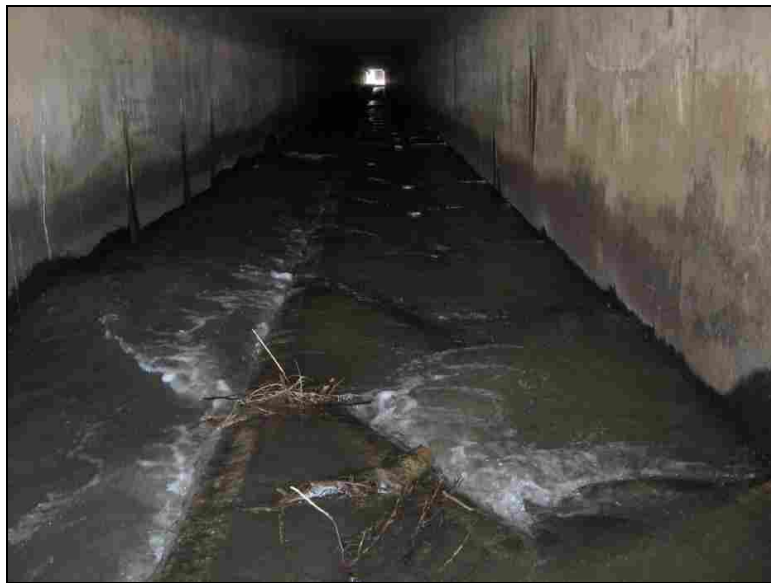
Figure 6-21: Orientation of Baffles in Diamond Fork #2 Culvert (Looking Downstream)
