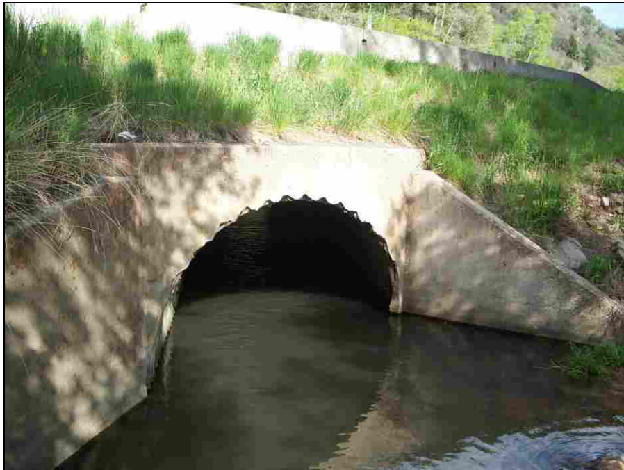
Figure 4-13: Outlet of Backwatered Culvert #3
