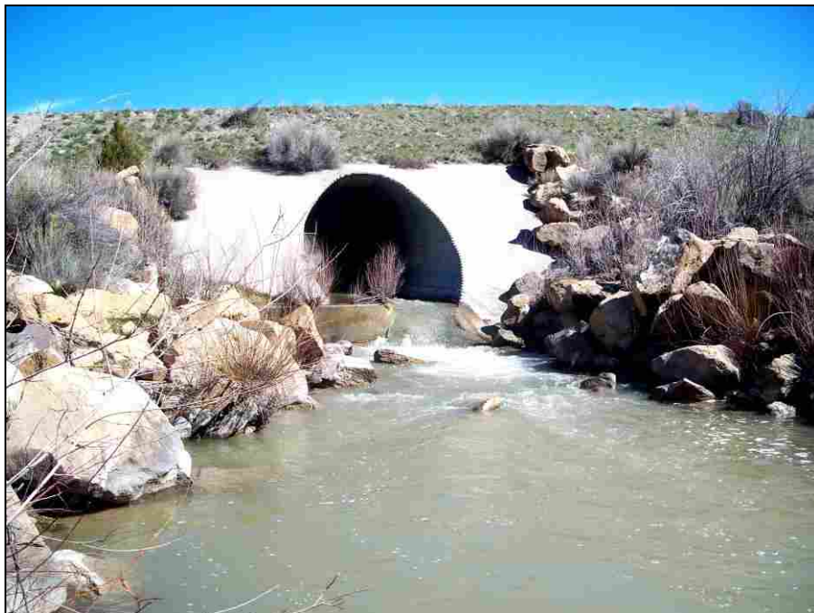
Figure 6-7: Salina Creek Culvert Outlet (Salina Creek Field Verification Site)
