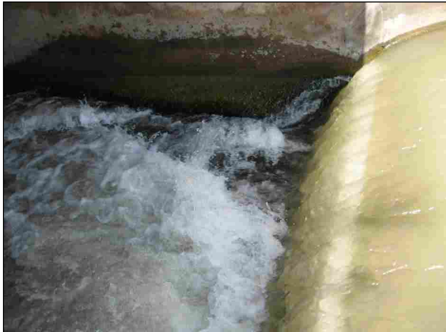
Figure 5-16: Detailed View of Spillway at Inlet
