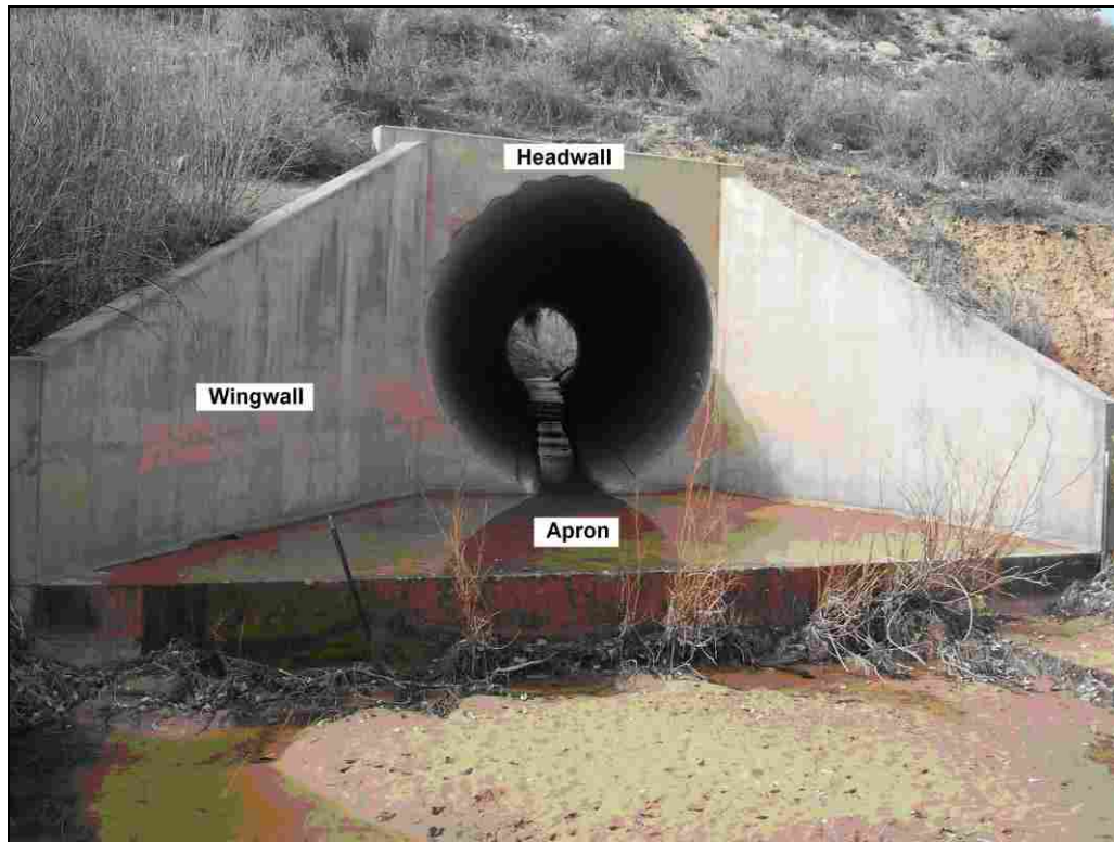
Figure 5-36: Culvert Headwall, Wingwalls and Apron
