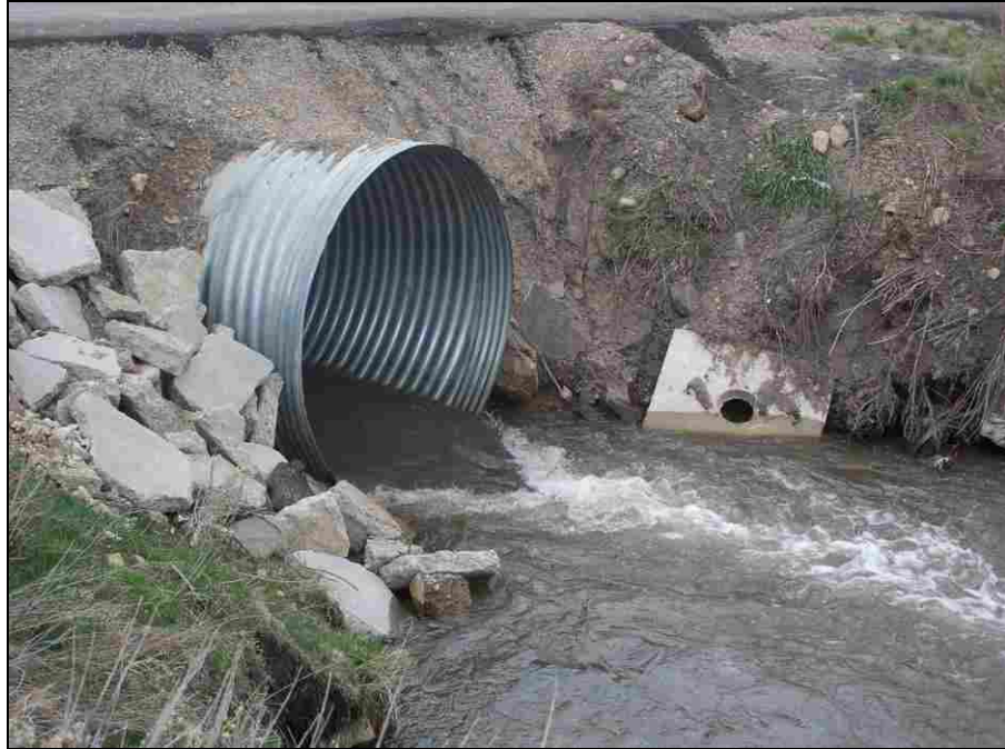
Figure 5-44: Hydraulic Jump Just Downstream of Outlet
