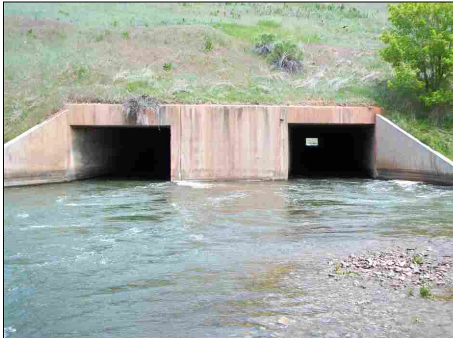
Figure 6-5: Diamond Fork Culvert #2 Outlet (Diamond Fork Field Verification Site)
