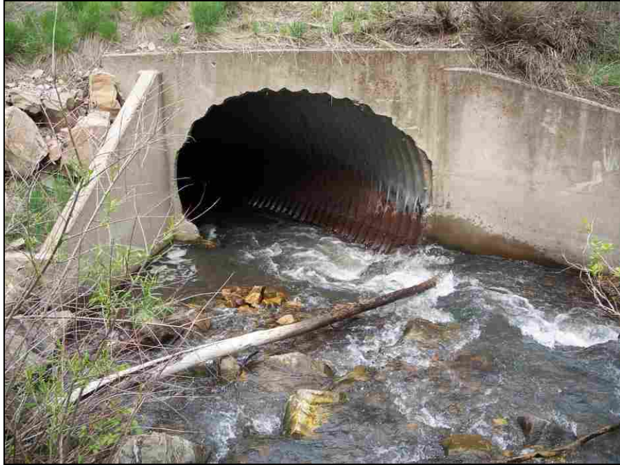
Figure 5-42: Hydraulic Jump Just Upstream of Inlet
