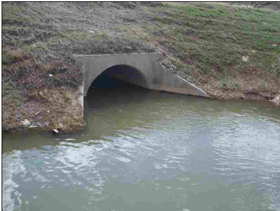
Figure 4-9: Outlet of Backwatered Culvert #1
