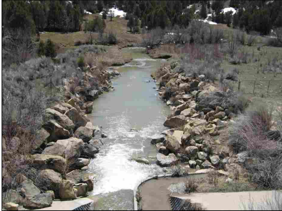
Figure 5-4: Additional Embankment Looking Downstream Photo Showing Floodplain
