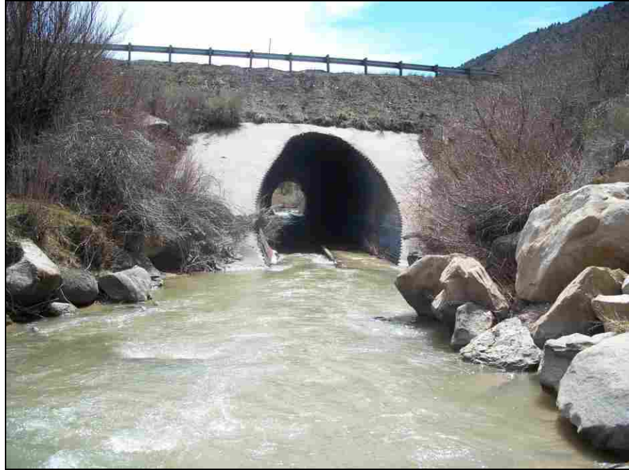
Figure 5-18: Photo of Inlet From 25 Feet
