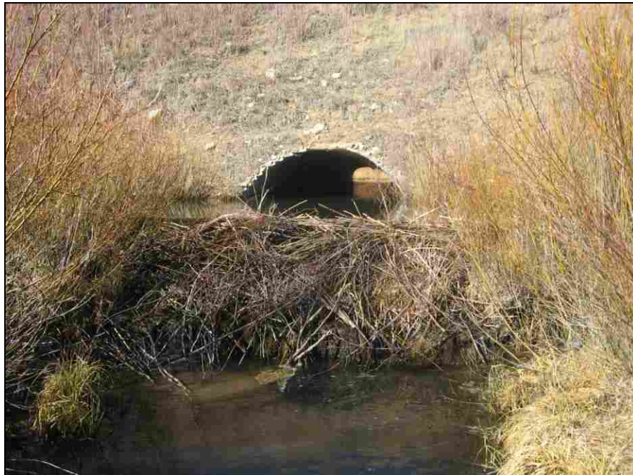
Figure 5-7: Beaver Dam Tailwater Control Relative to the Culvert Outlet
