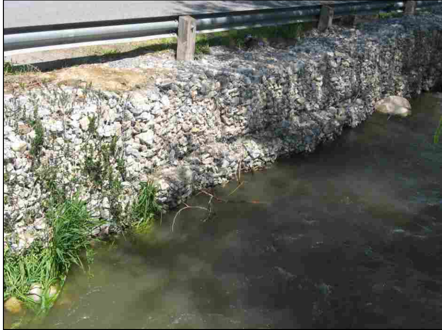
Figure 5-24: Gabion Wall
