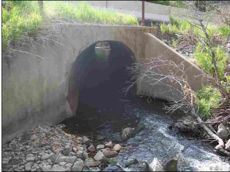
Figure 6-12: Daniel's Creek Culvert #1 Inlet (Daniels Creek Field Verification Site)
