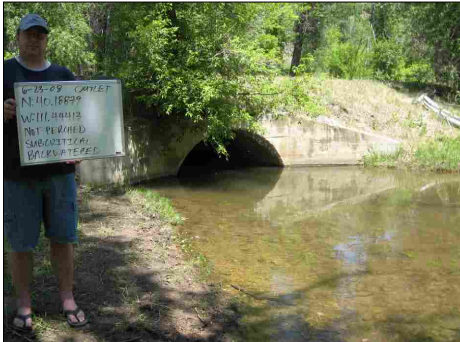
Figure 4-2: Hydraulic Evaluation Photo Taken at the Outlet
