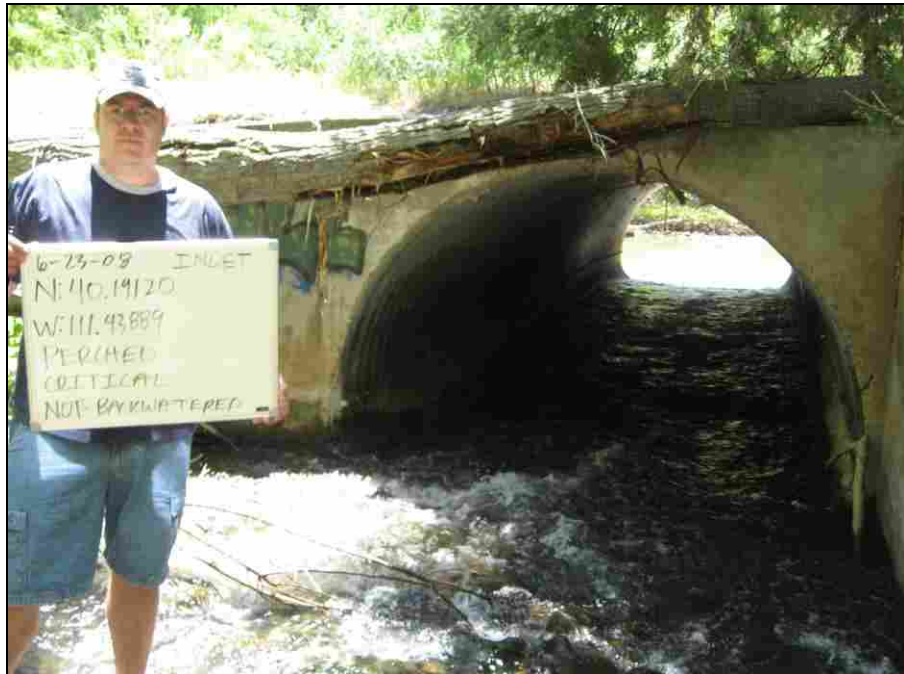
Figure 3-6: Hydraulic Evaluation Photo of a Culvert Inlet
