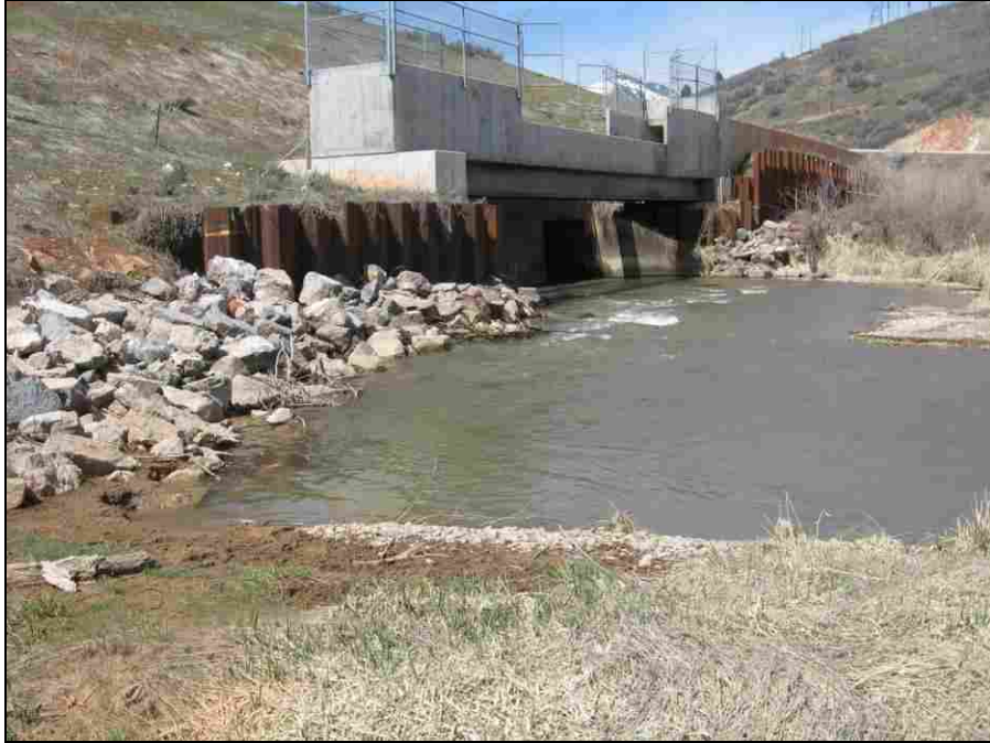
Figure 5-22: Riprap and Sheet Pile Near Inlet
