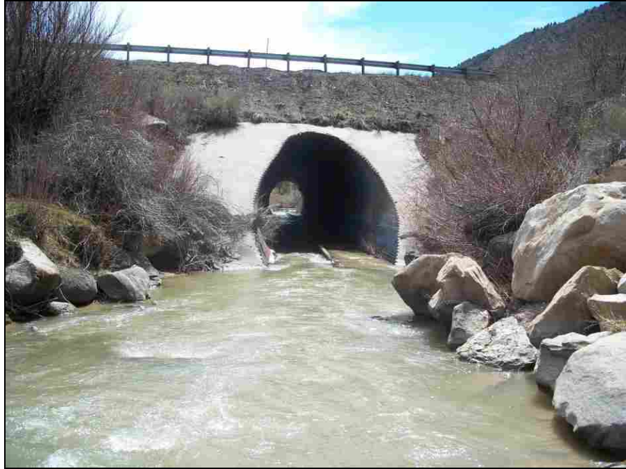
Figure 6-8: Salina Creek Culvert Inlet (Salina Creek Field Verification Site)
