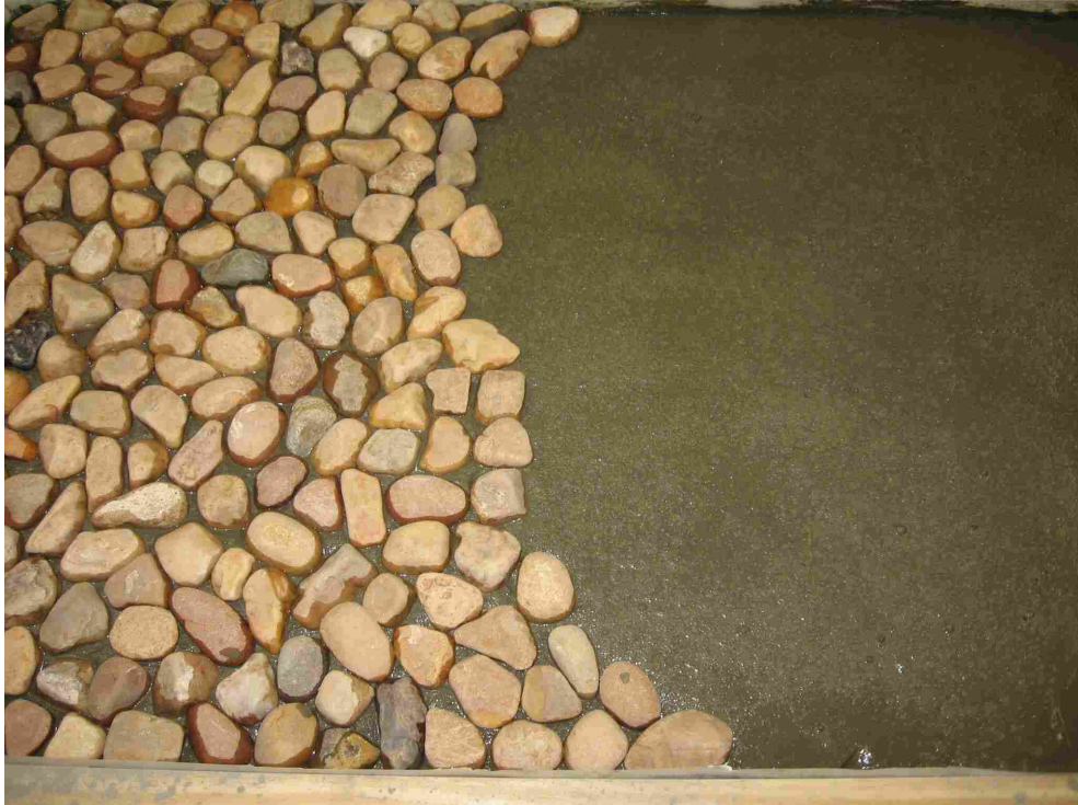
Figure B.5: Placing gravel in the frame
