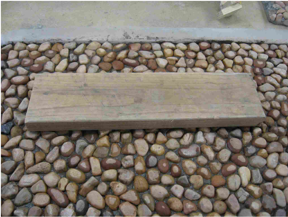
Figure B.6: Tamping the gravel
