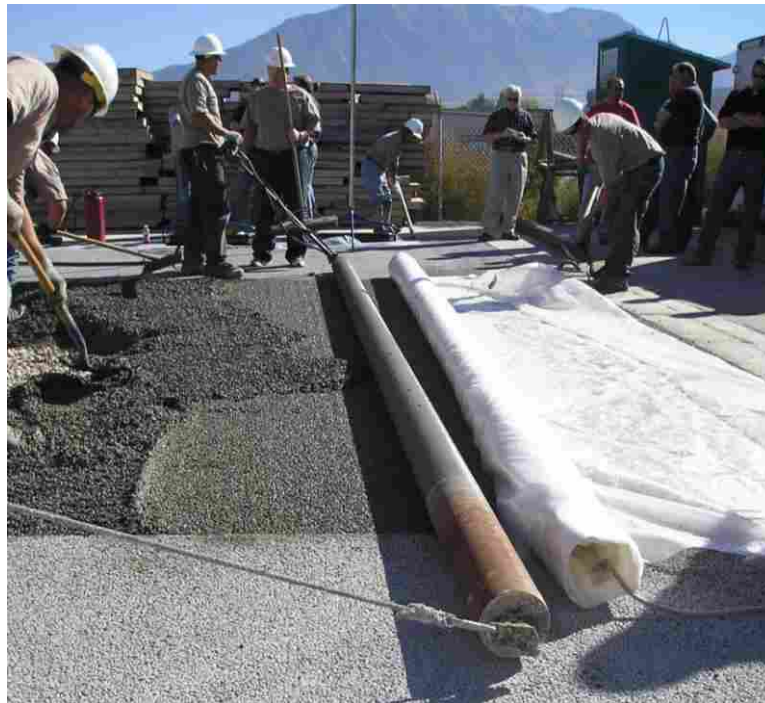
FIGURE 2.1 Steel roller used for consolidation.
