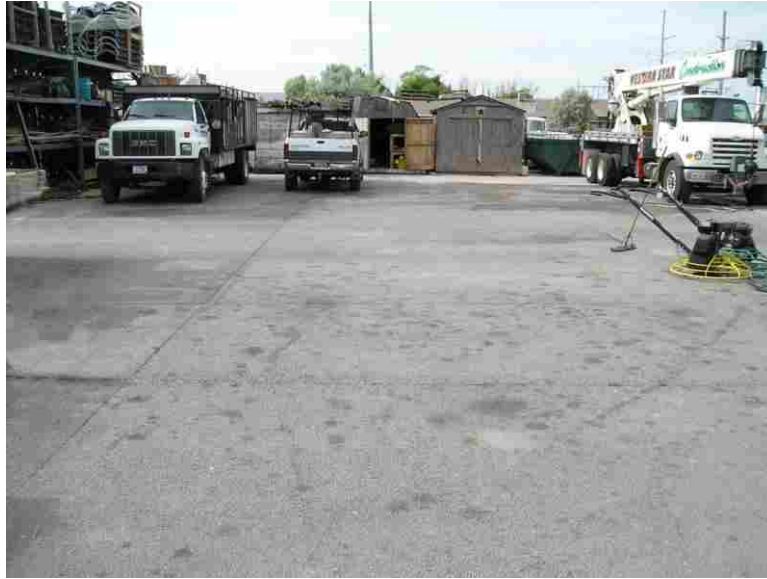
FIGURE 3.10 Pervious concrete test slab in Orem, Utah.
