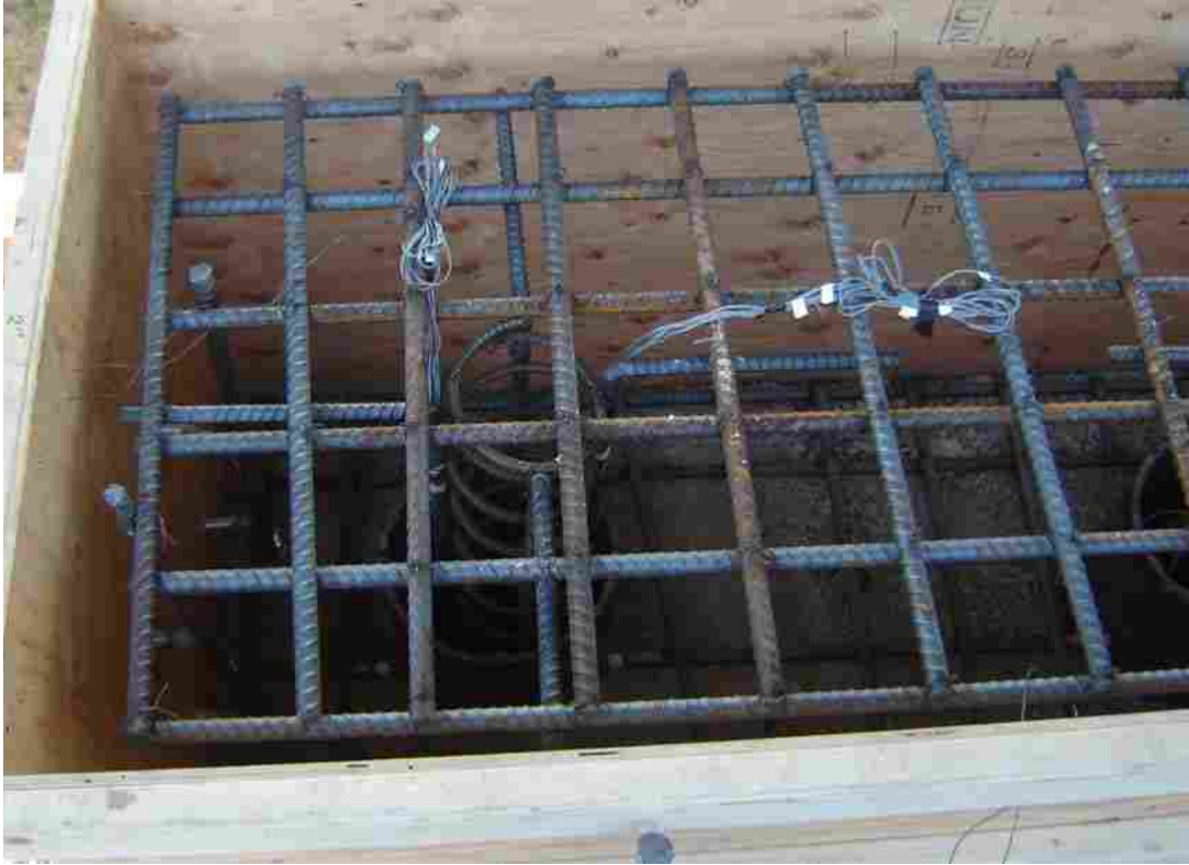
Figure 3-13 Photograph of Pile Cap 1 reinforcing.
