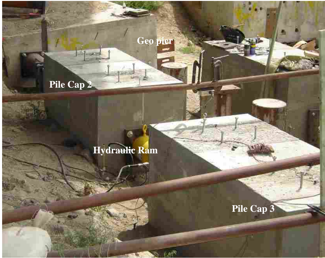
Figure 3-18 Photograph of equipment arrangement for test on Pile Cap 3.
