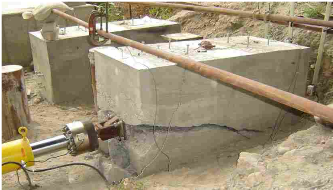
Figure 5-14 Test Cap 3 at failure.
