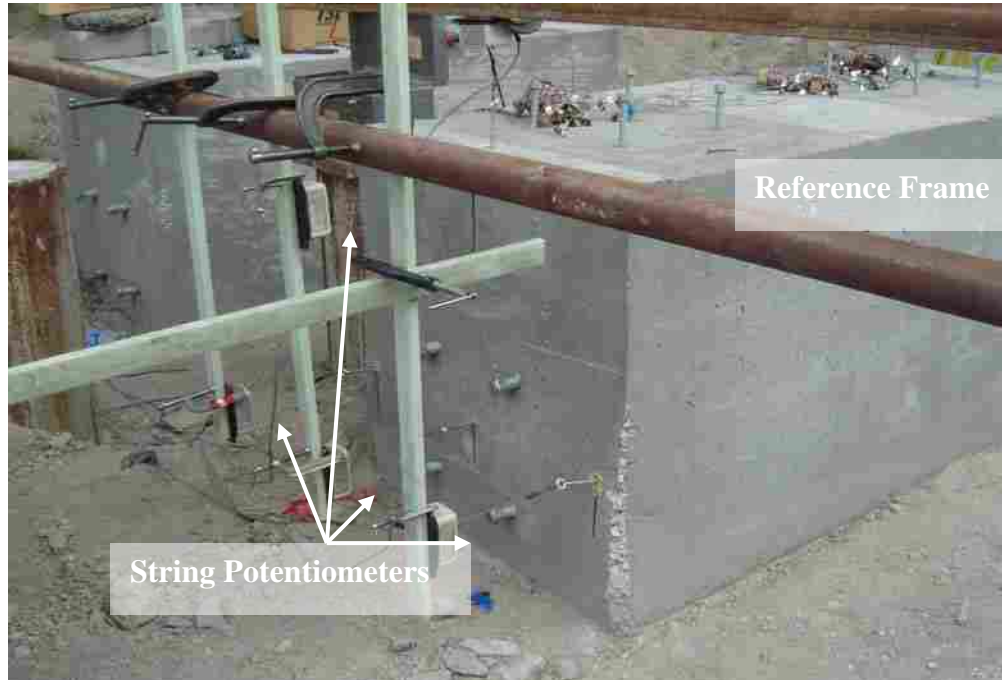
Figure 3-10 Photograph of string potentiometers setup (typical all caps).
