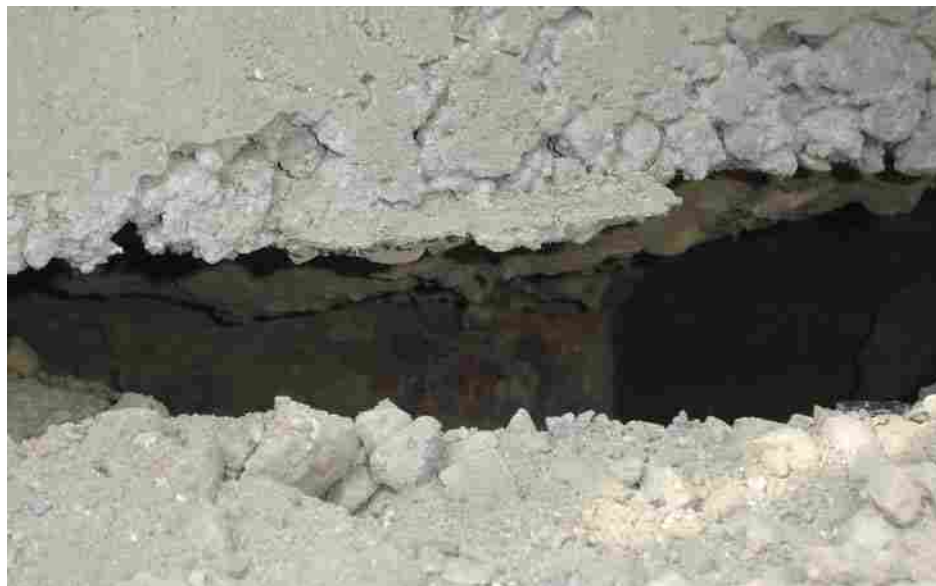
Figure 5-11 Test Cap 2 failure in pullout.
