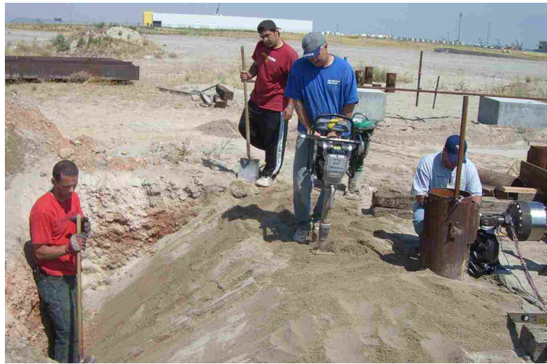
Figure 3.7 Photograph of Soil Compaction During Test Three.
