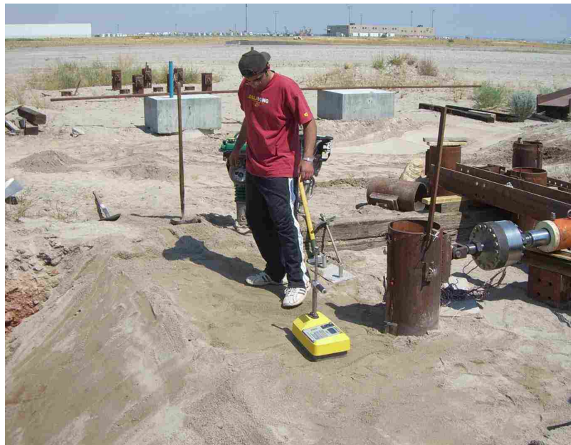
Figure 3.8 Photograph of Nuclear Density Testing During Test Three.
