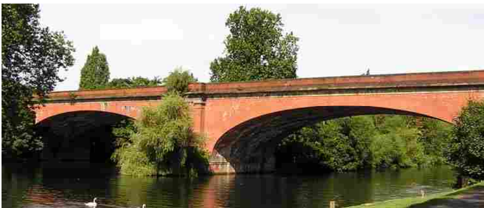
Figure 2-5 – The Sounding Arch Bridge in Maidenhead, England
