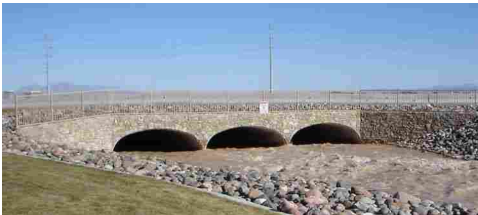
Figure 2-12 – A Hydro-Arch bridge in Las Vegas, Nevada
