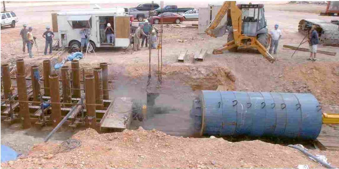
Figure 1.1: Lateral Statnamic testing (S.R. Johnson, 2003a).
