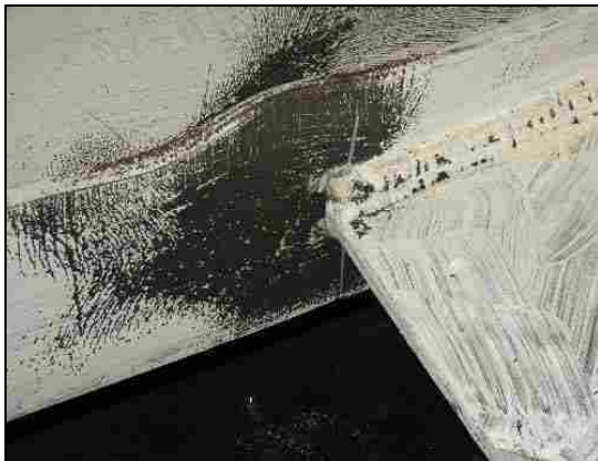
(c) Fracture of Beam
