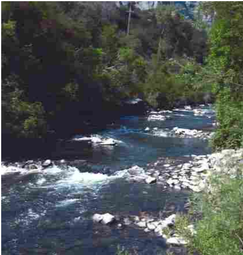
Figure 2-4. Bendway Weirs on the Provo River.
