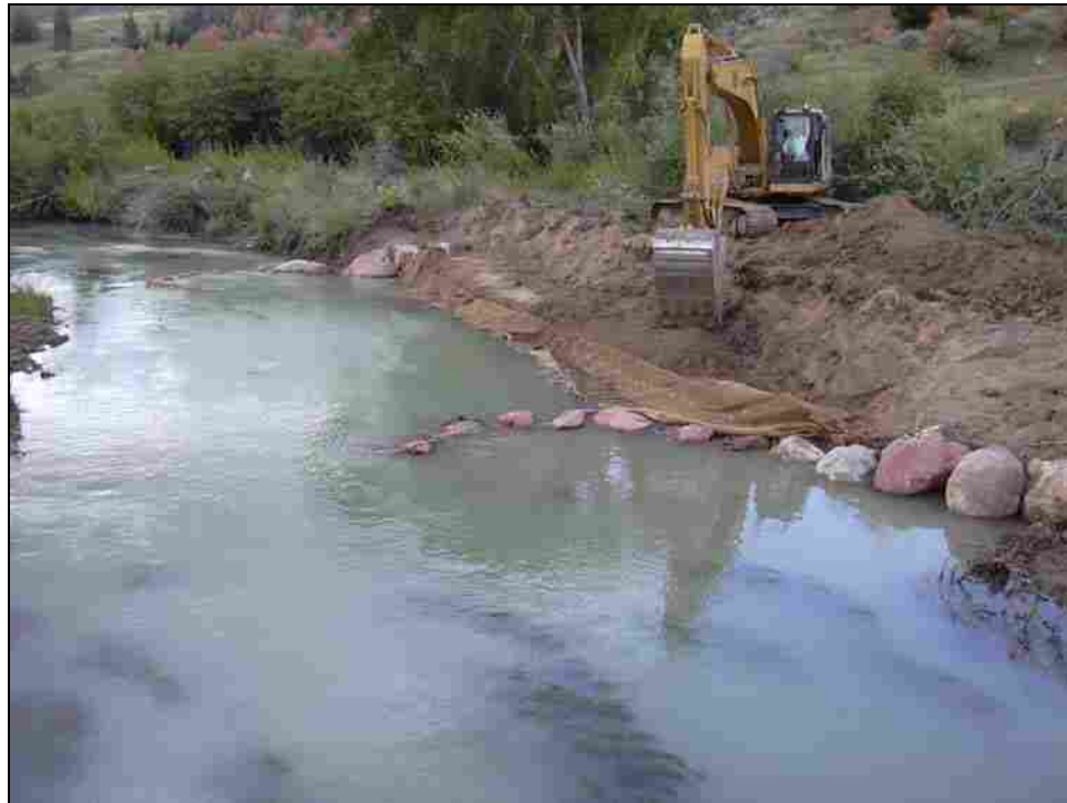
Figure 3-6. View of Construction From Bridge.
