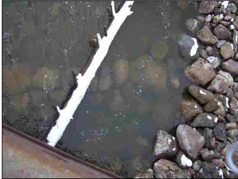
Figure 4-21. Bendway Weir on the North Fork Provo River Just After Installation.
