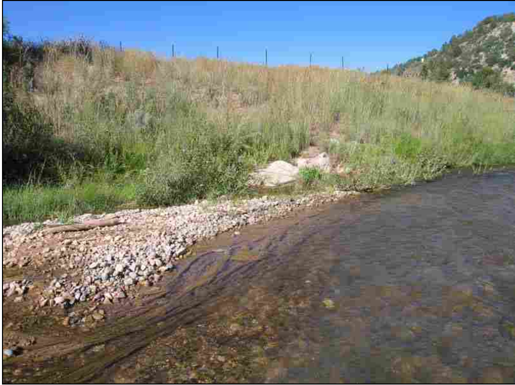
Figure 4-29. J-Hook at Thistle Creek After Runoff.
