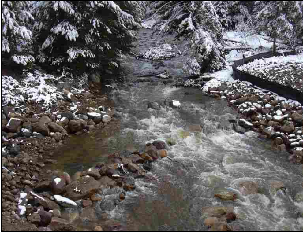
Figure 2-1. Drop Structure on the North Fork of the Provo River.
