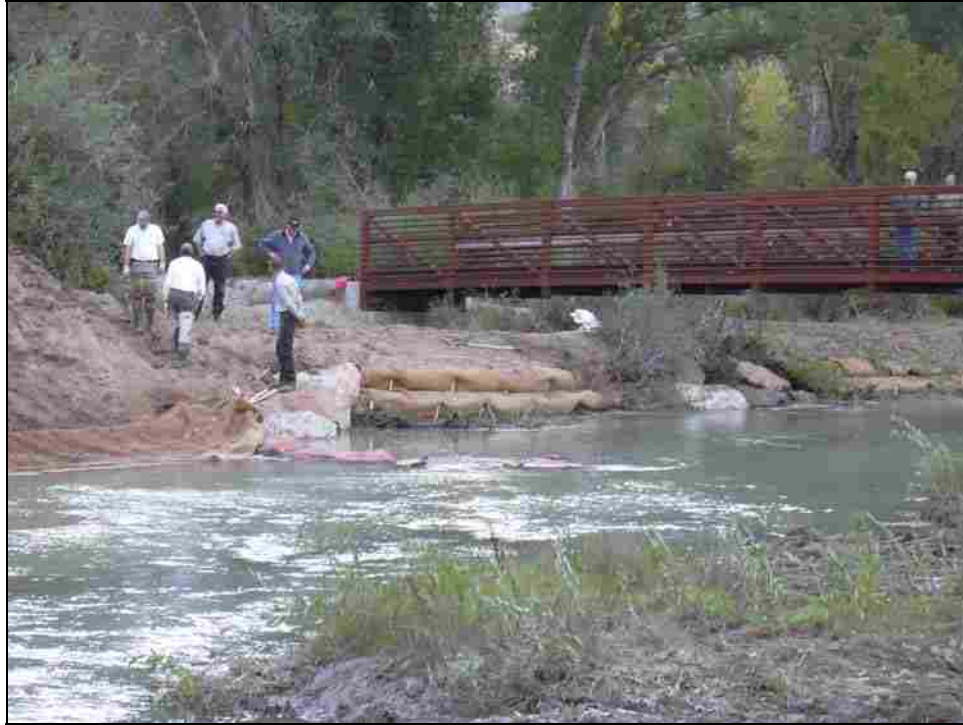
Figure 3-5. View of Construction of Structure Near Footbridge.
