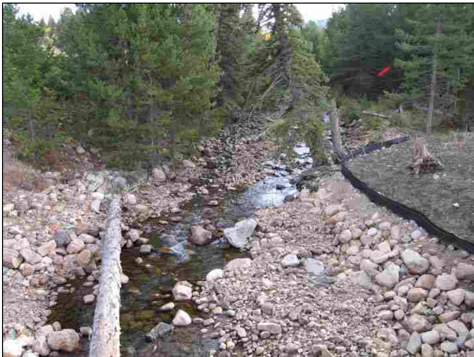
Figure 4-24. Weir Site on the North Fork Provo River After Runoff.
