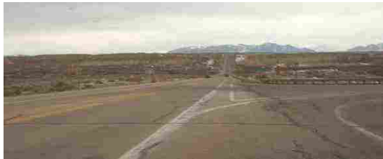
(a) Intersection of US-6 and SR-136
