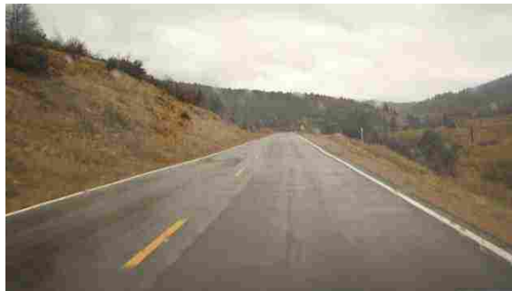
(a) MP 2, Eastbound
