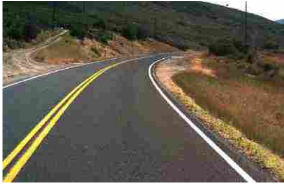
(a) MP 1, Eastbound
