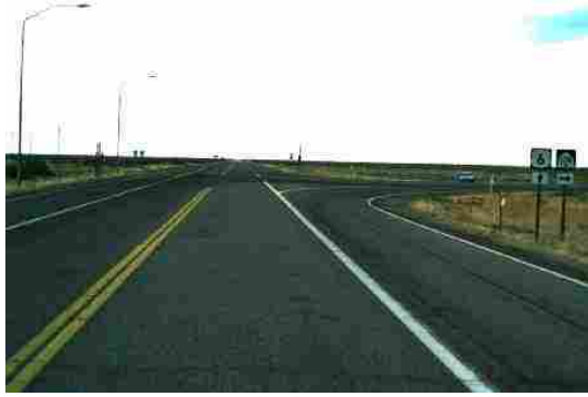
(a) Intersection of US-6 and SR-174
