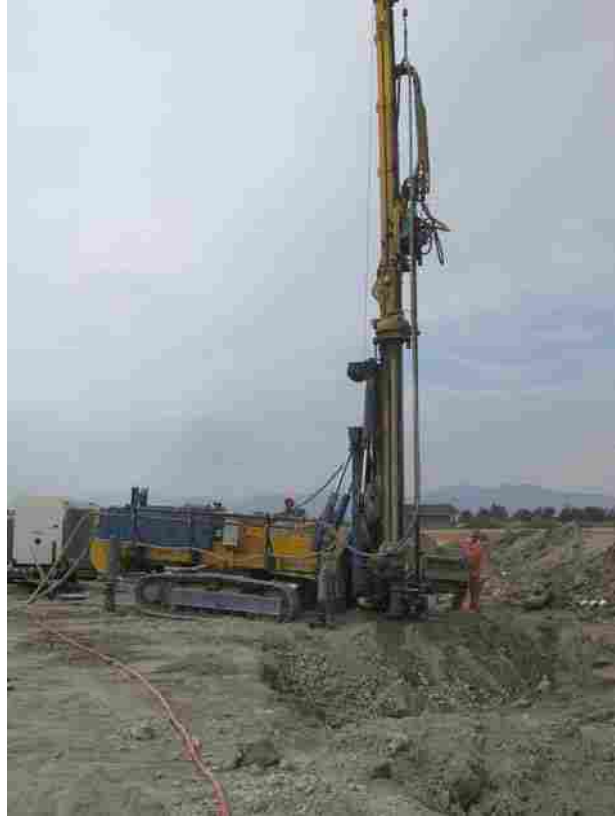
Figure 5-1 Photo of drill rig in position above buried foundation.
