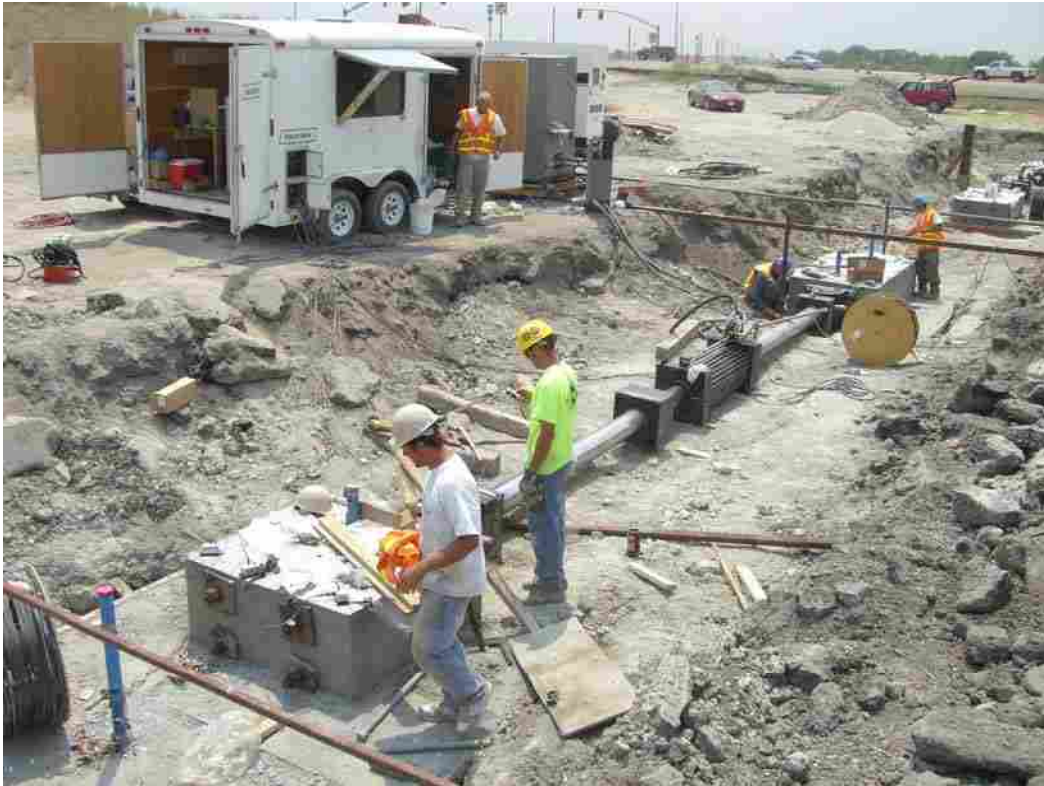
Figure 4-10 Photo of actuator setup between caps 1 & 2.
