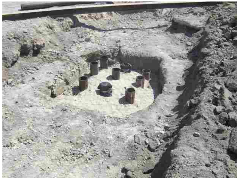
Figure 4-2 Driven pile layout prior to cap construction.
