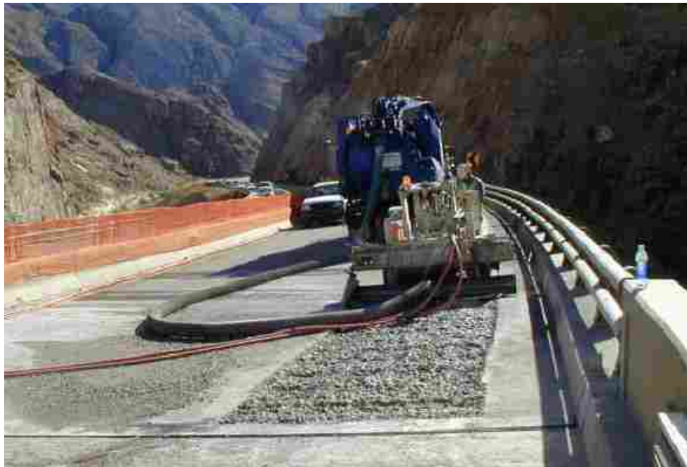
FIGURE 2.3 Removal of concrete by hydrodemolition (18).
