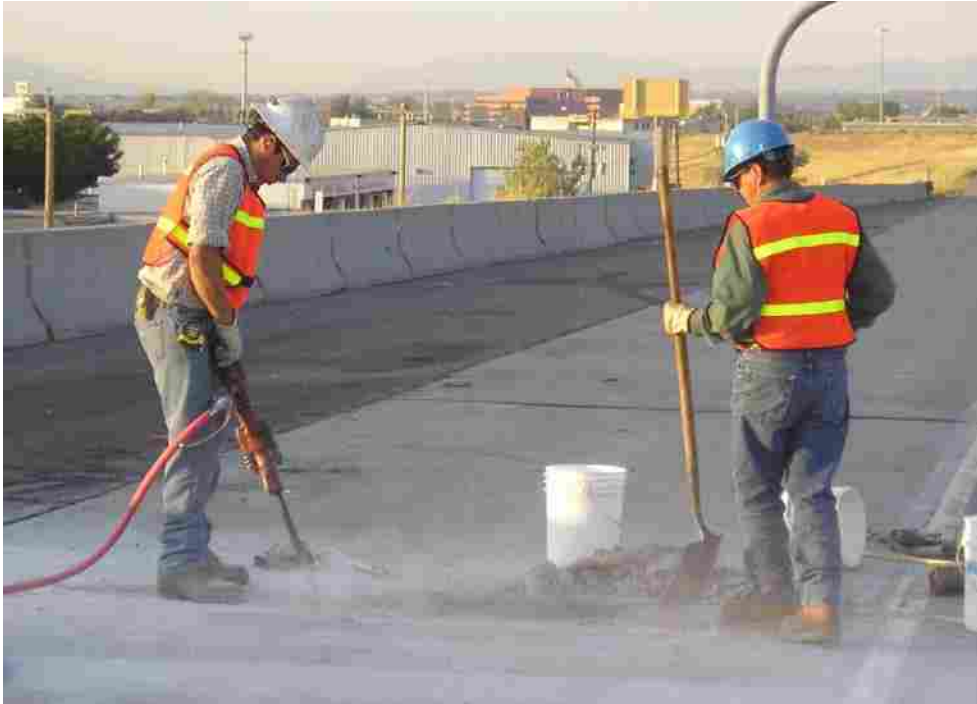
FIGURE 2.4 Removal of concrete by jackhammering.
