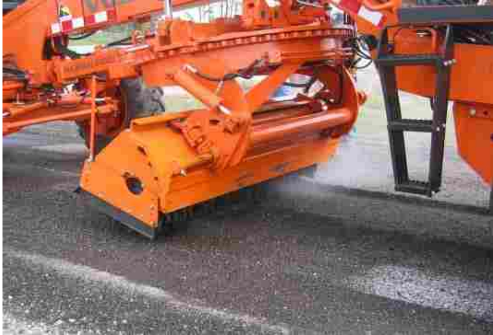
FIGURE 2.2 Removal of asphalt by milling machine (17).
