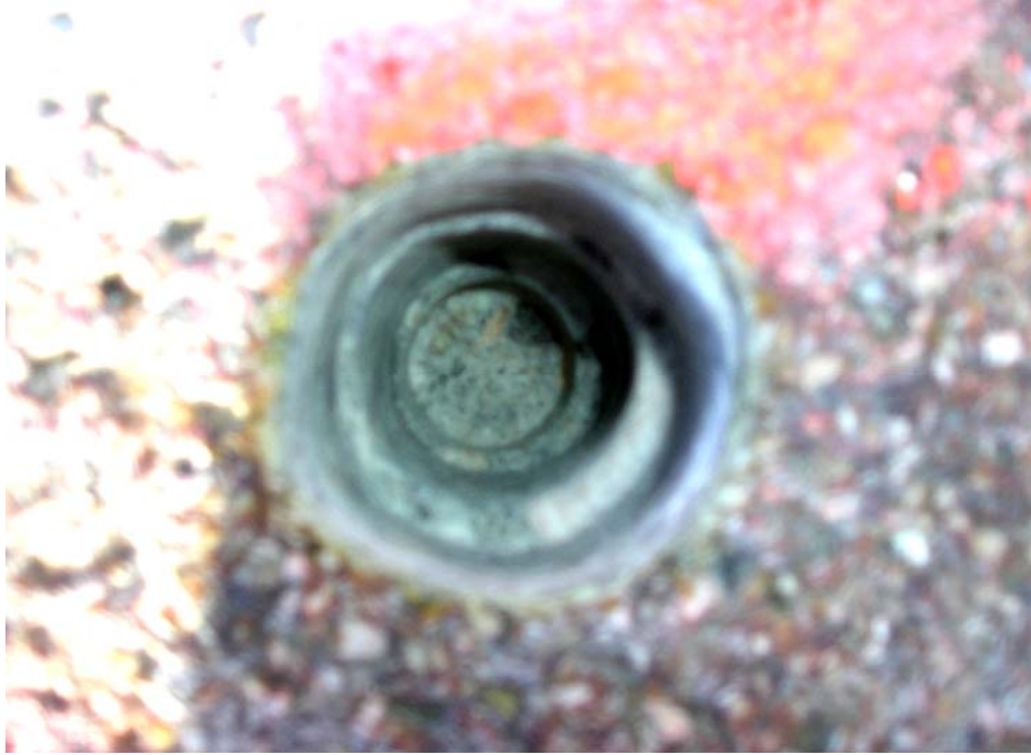
FIGURE 3.5 Example of a typical hole after drilling.
