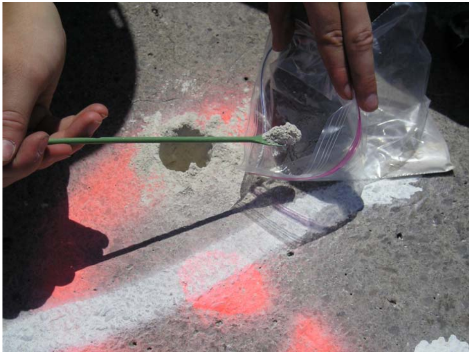
FIGURE 3.6 Removal of pulverized concrete from drilled hole.
