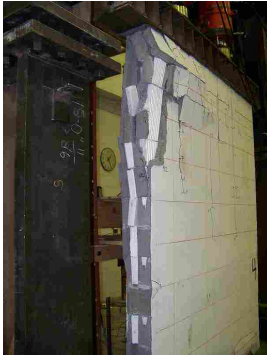
Side View at Failure (wall #4)
