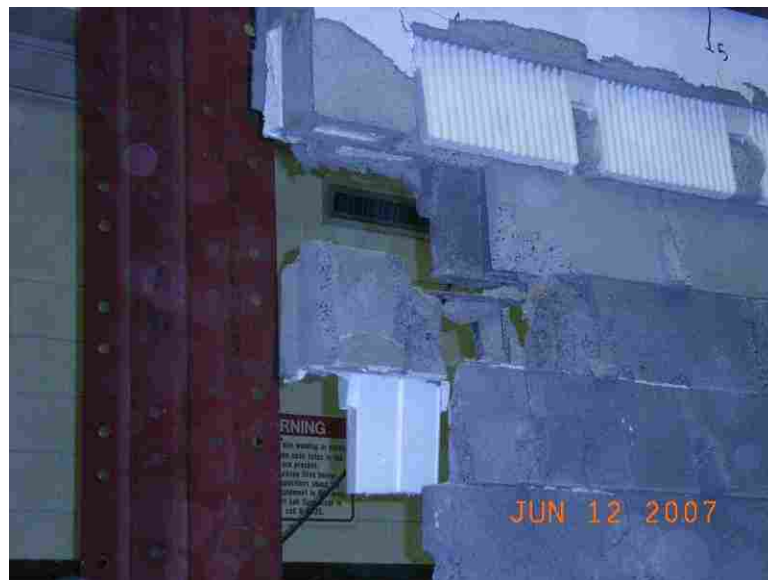
Close-up of East end of Wall at Failure (wall #8)
