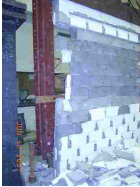
Figure 6.5 Wall #8 at Failure
