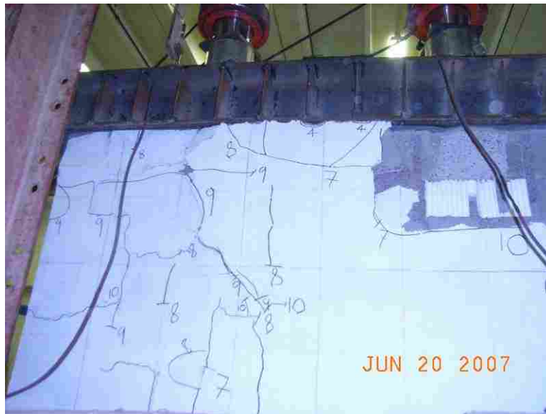
Close-up of Failed Exterior Section (wall #6)
