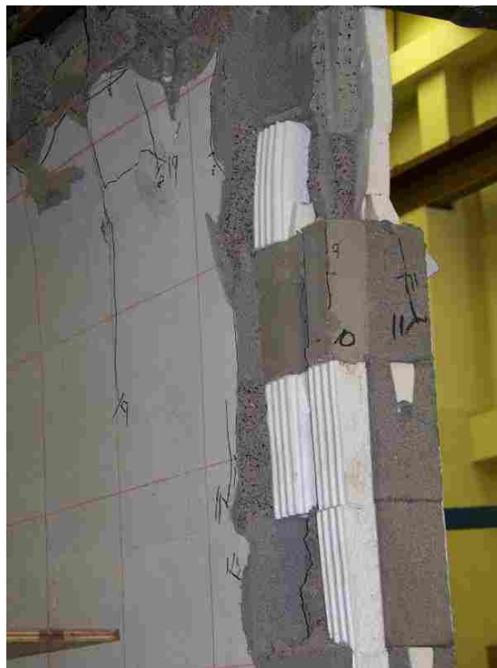
Close-up View of Failed Section (wall #3)
