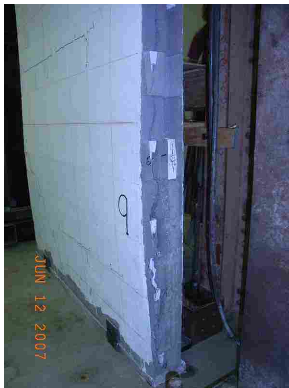
Vertical Cracking in Sides of Wall (wall #9)
