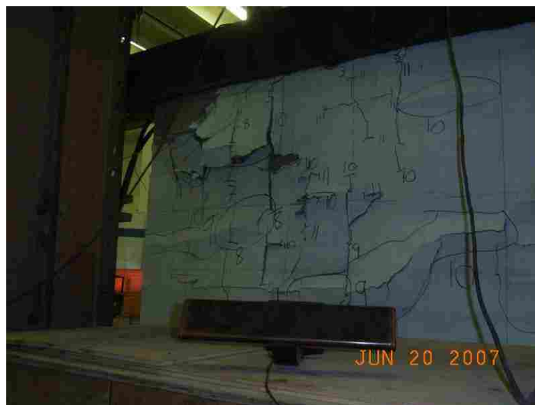
Failure at Exterior Side of Wall (wall #7)
