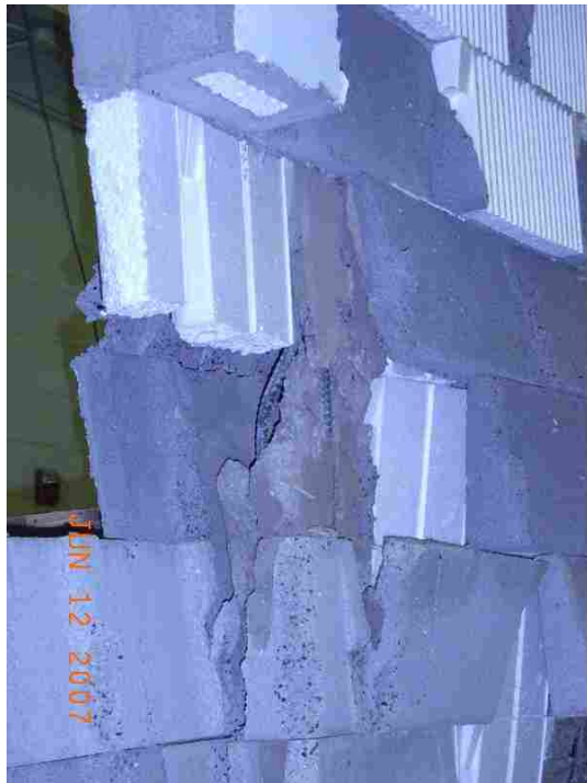
Rebar Buckling at Failure (wall #9)
