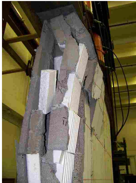
Close-up View of Failed Section (wall #4)
