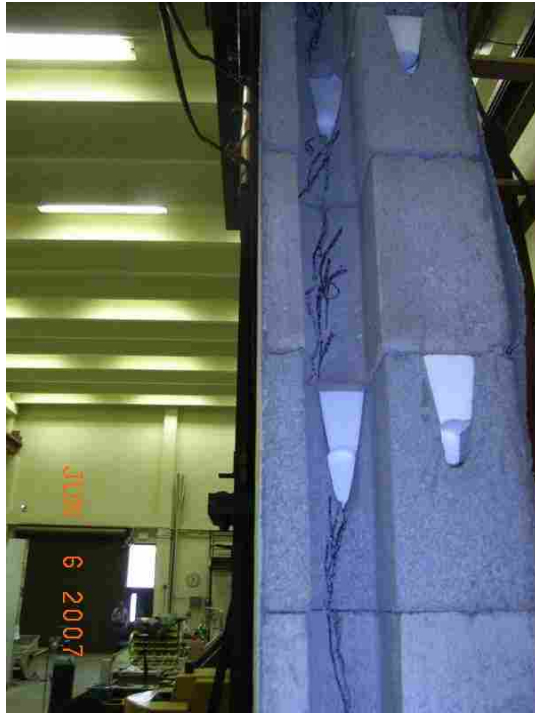
Vertical Cracks in Sides of Wall (wall #10)
