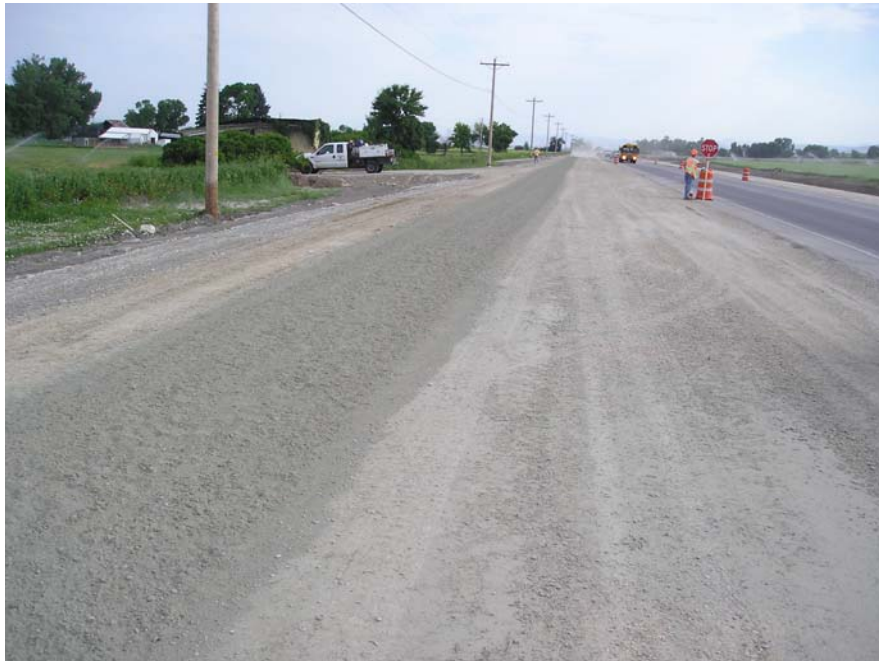
FIGURE 3.6 US-91 site picture.
