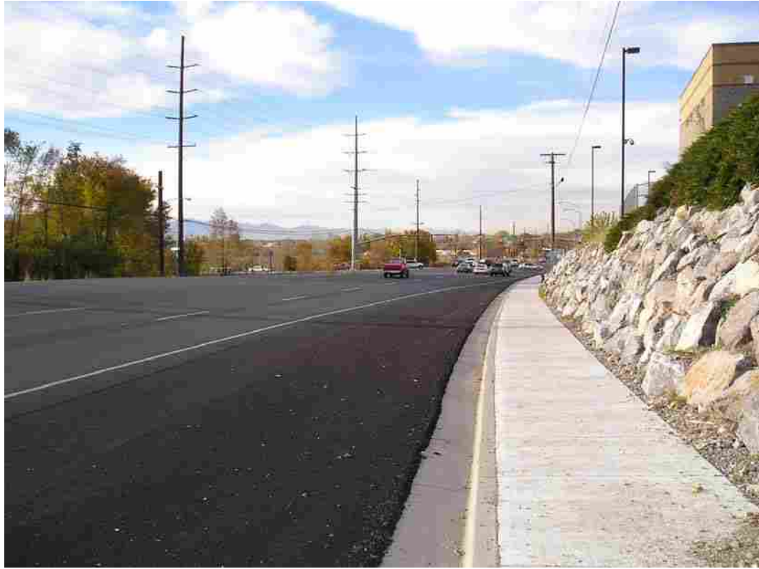
Figure 4.18 Intersection of S.R. 89 & 1860 South in Provo.
