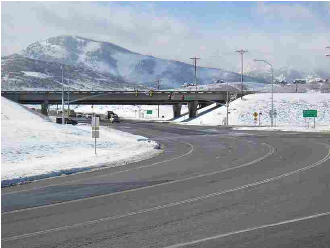
Figure 4.9 Intersection of S.R. 248 & S.R. 40 near Park City.
