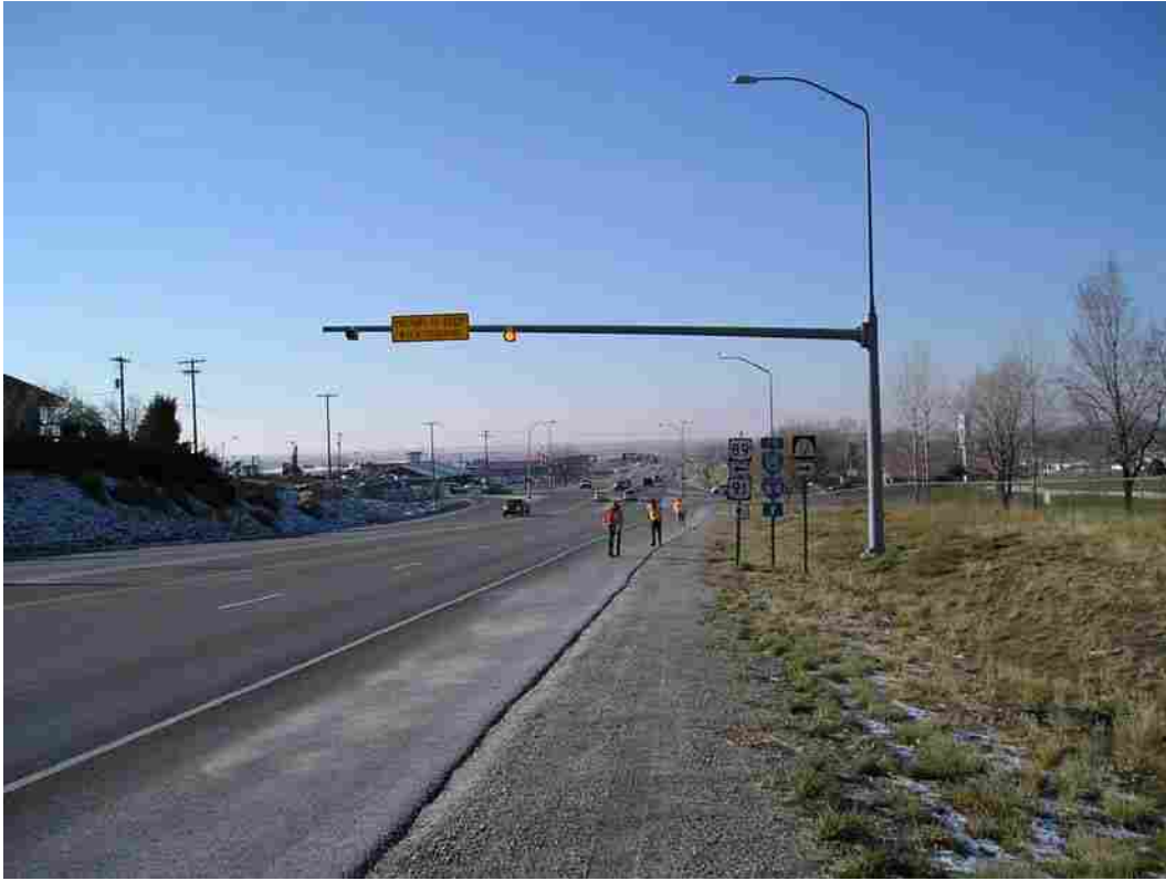
Figure 4.3 Intersection of S.R. 91 & Main Street in Brigham City.
