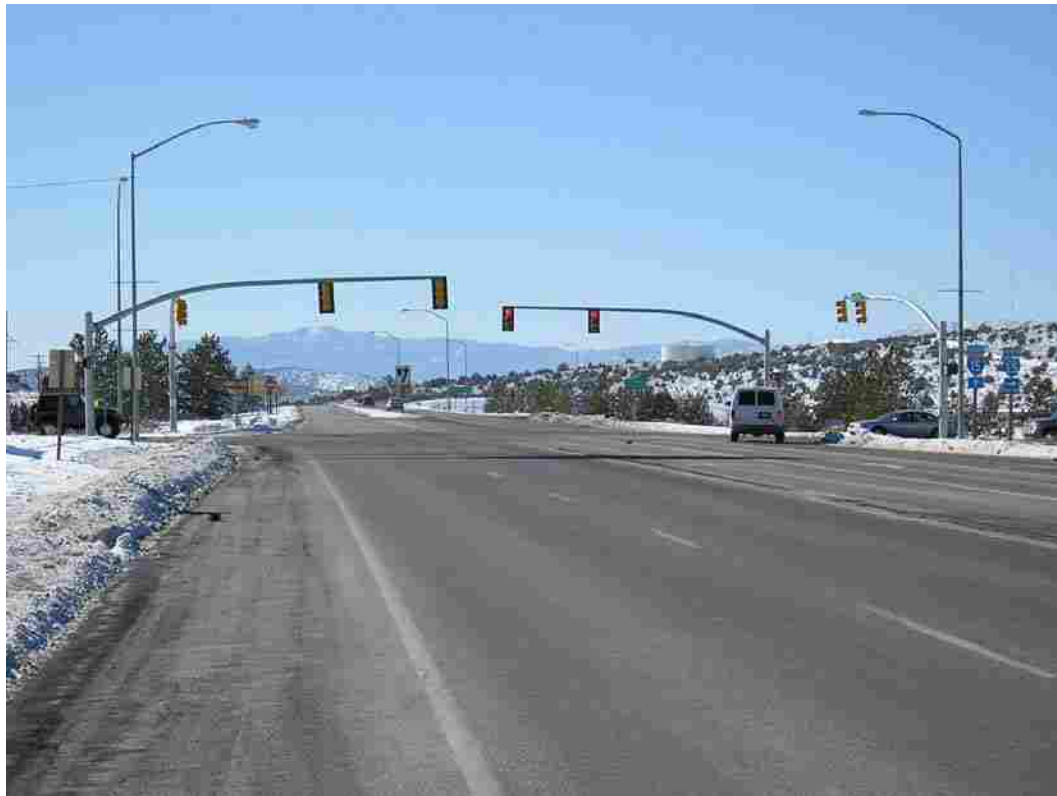
Figure 4.20 Intersection of S.R. 130 & Cross Hollow in Cedar City.
