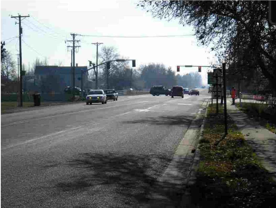
Figure 4.7 Intersection of S.R. 126 & S.R. 134 in Farr West.
