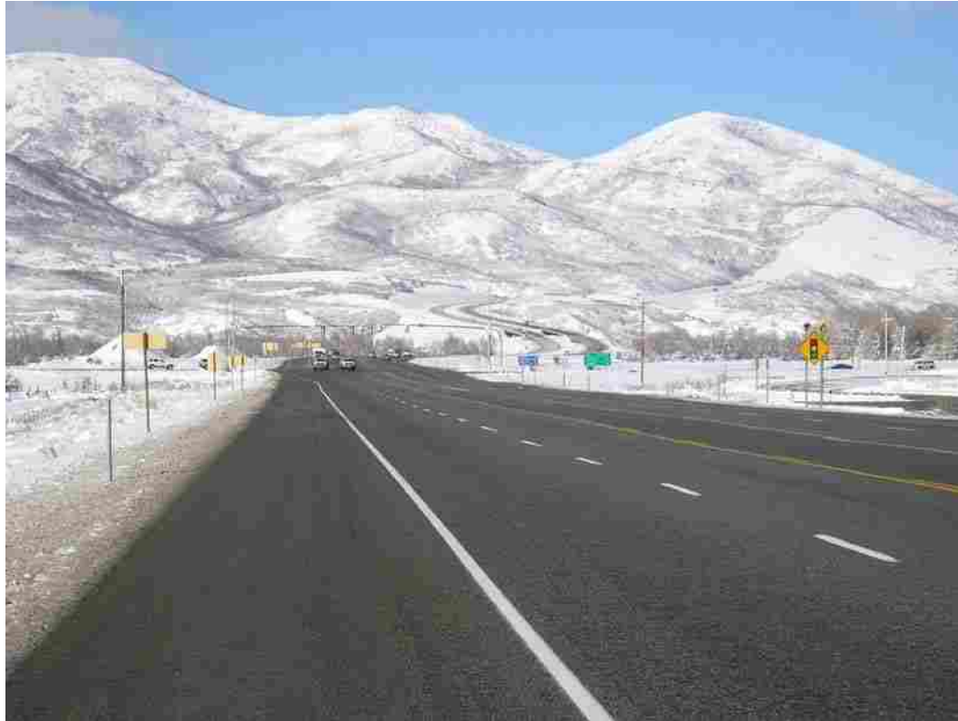
Figure 4.16 Intersection of S.R. 40 & S.R. 32 in Heber.
