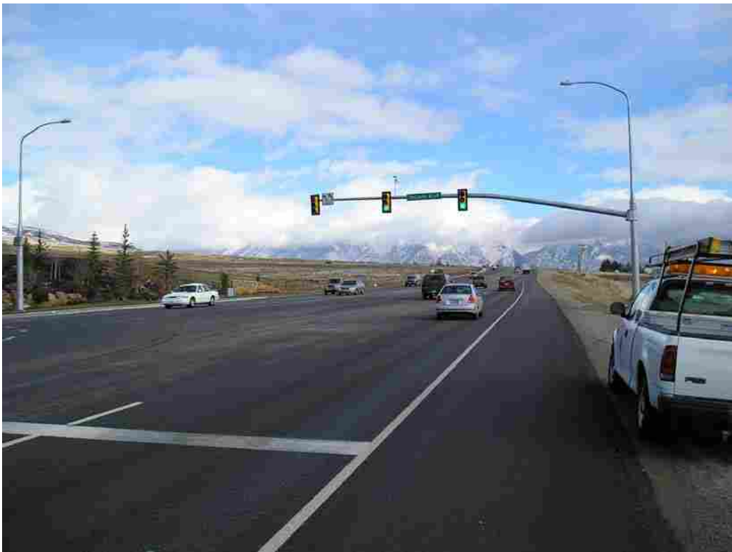
Figure 4.13 Intersection of S.R. 92 & Triumph Boulevard in Lehi.
