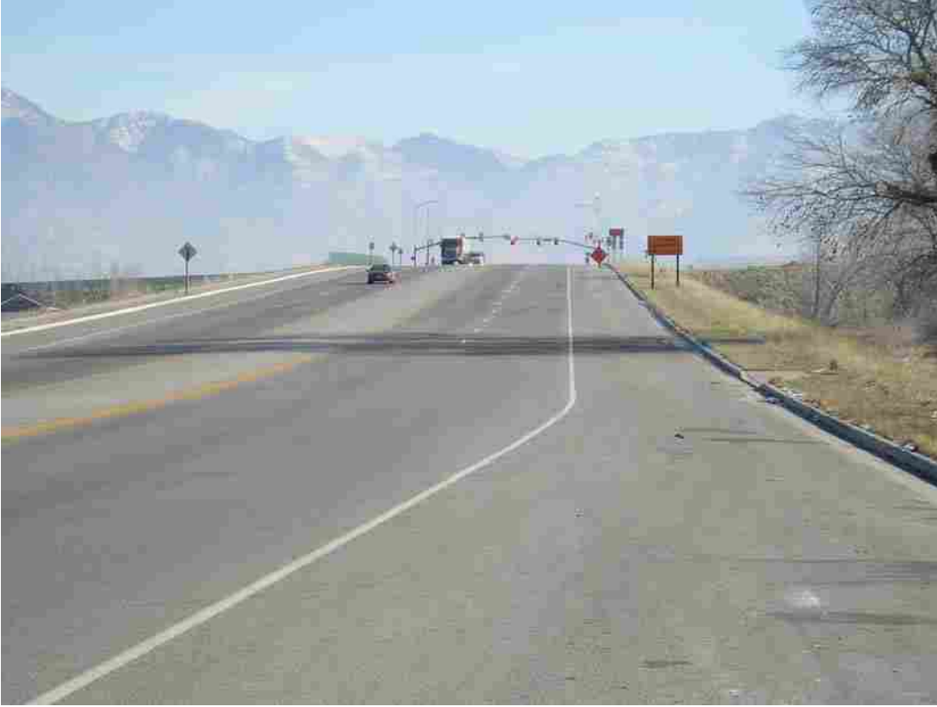
Figure 4.5 Intersection of S.R. 39 & S.R. 126 in Marriot-Slaterville.
