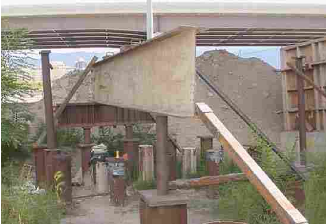
Figure 4.6 Static Load Test Frame (2004 Static Load Tests)
