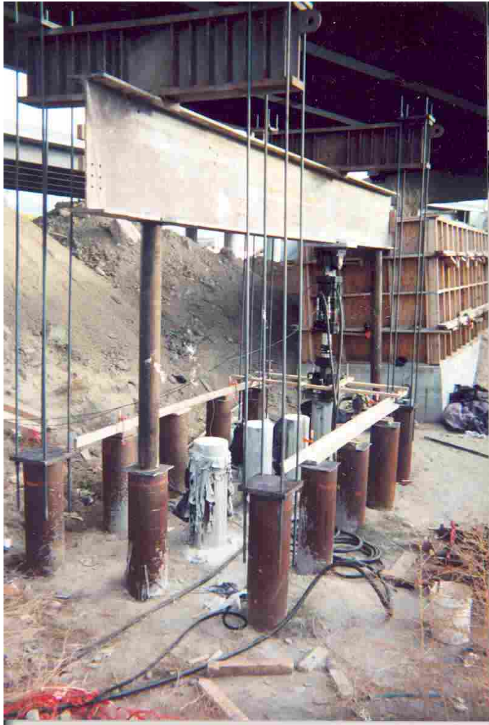
Figure 4.5 Static Load Test Frame (2002 Static Load Tests)
