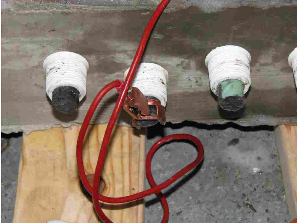
FIGURE 3.11 Electrical connection to rebar.
