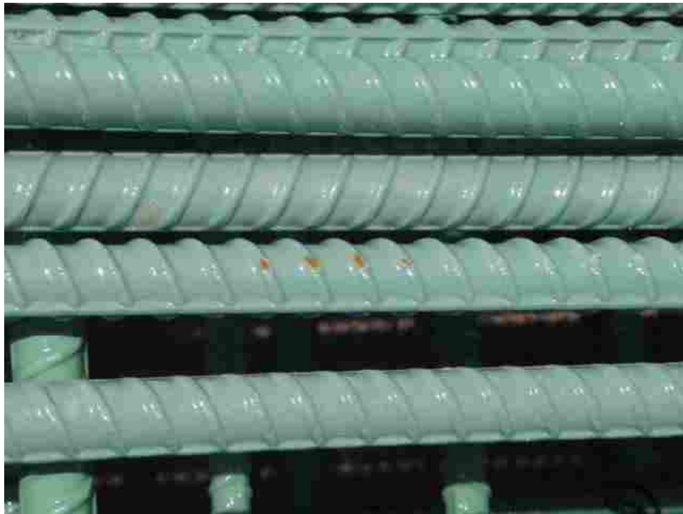
FIGURE 2.3 Rib scrape damage in the field.
