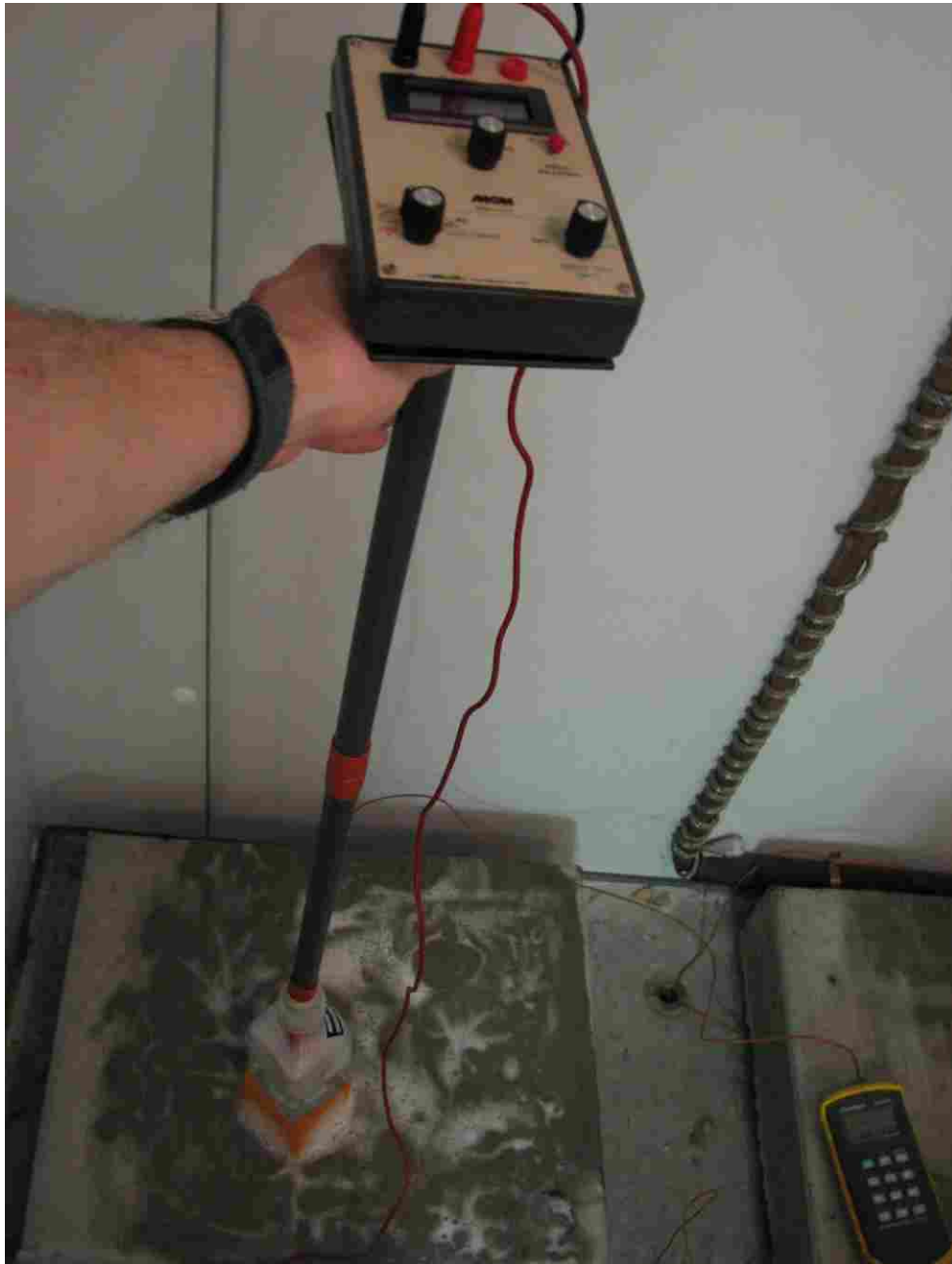
FIGURE 3.13 Half-cell potential testing.
