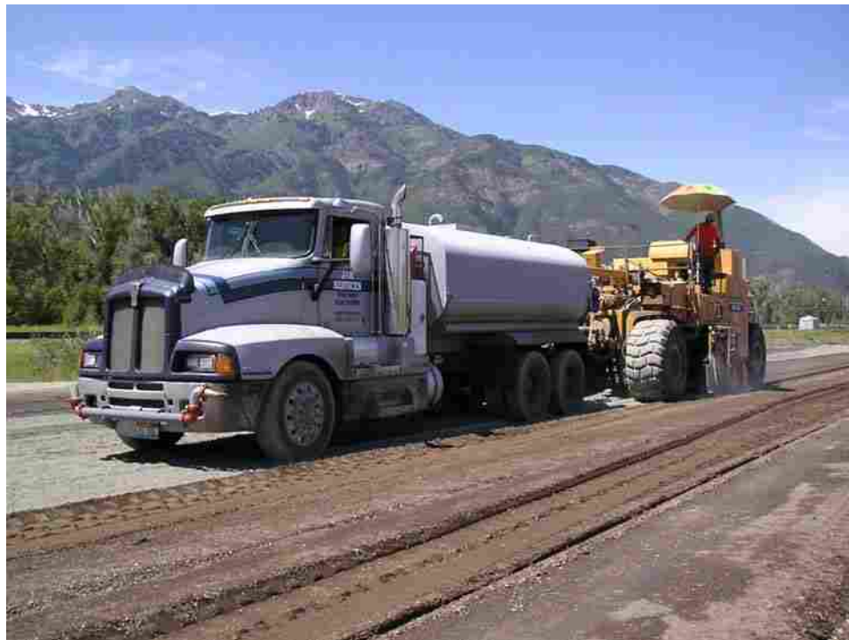
FIGURE 3.3 Reclaimer with water truck.
