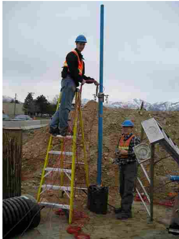
Figure 4-8 Installing Pipe Sections One at a Time at Redwood Road and SR-201 (author photo)
