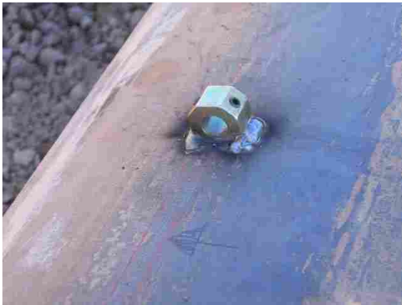
Figure 4-3 End Block after being Welded to the Pile
