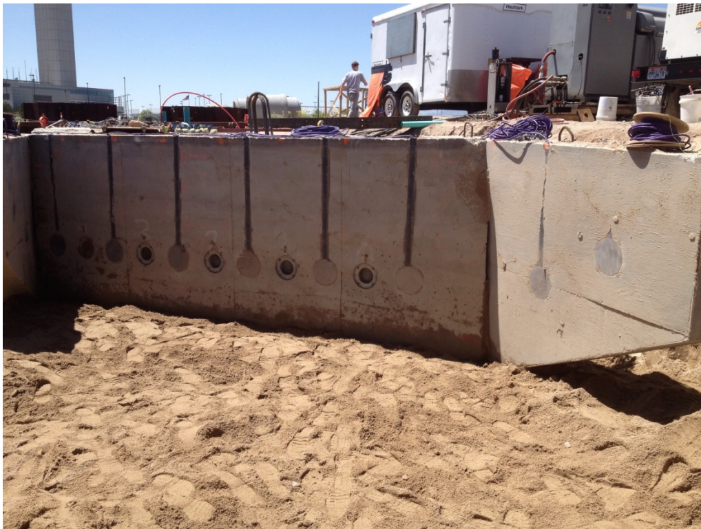
Figure 3.11. Geokon® pressure cell layout for 45° skew test (Smith 2014).
