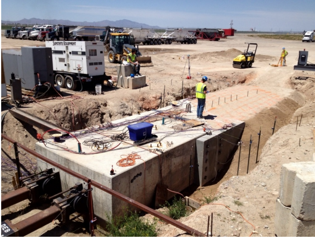
Figure 3.10. Compacted backfill for 45° skewed abutment.
