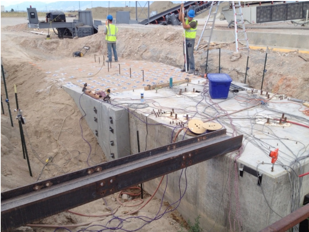
Figure 3.9. Compacted backfill for the non-skewed abutment.
