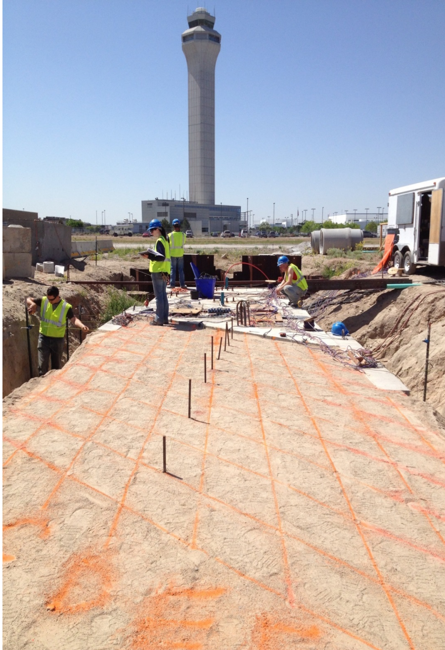
Figure 3.13. Spray-painted grid for 45° skew (Smith 2014).
