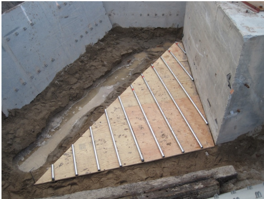
Figure 3.6. Steel rollers used to reduce friction at the base of the wedge sections.
